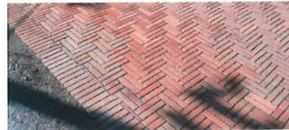
'PLANK' STYLE BRICK PAVER (PERMEABLE)
