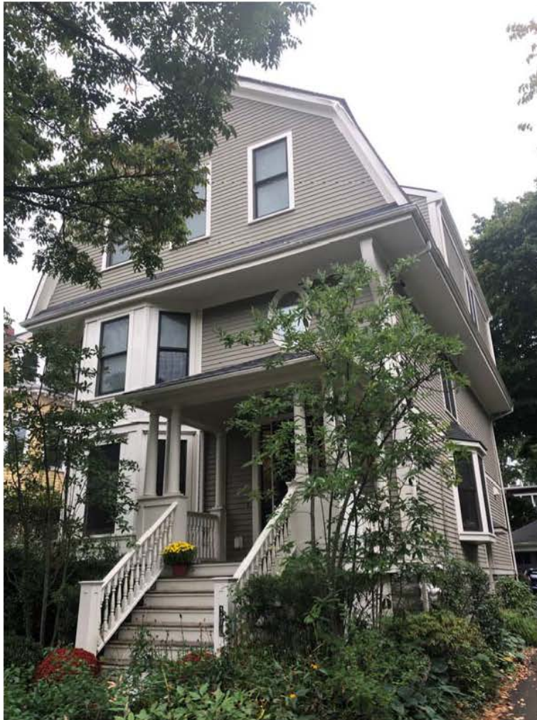
Existing Front of House; to remain as is
