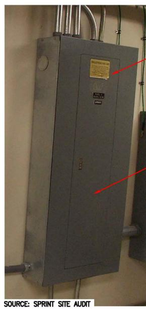
EXIST. 200A-2P MAIN CIRCUIT BREAKER (MCB) WITHIN EXIST. CIRCUIT BREAKER
