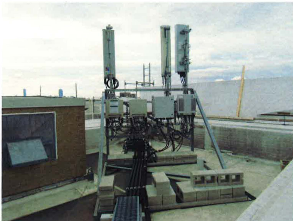
Photo 2: Sample photo illustrating the existing beta sector ballast frame.
