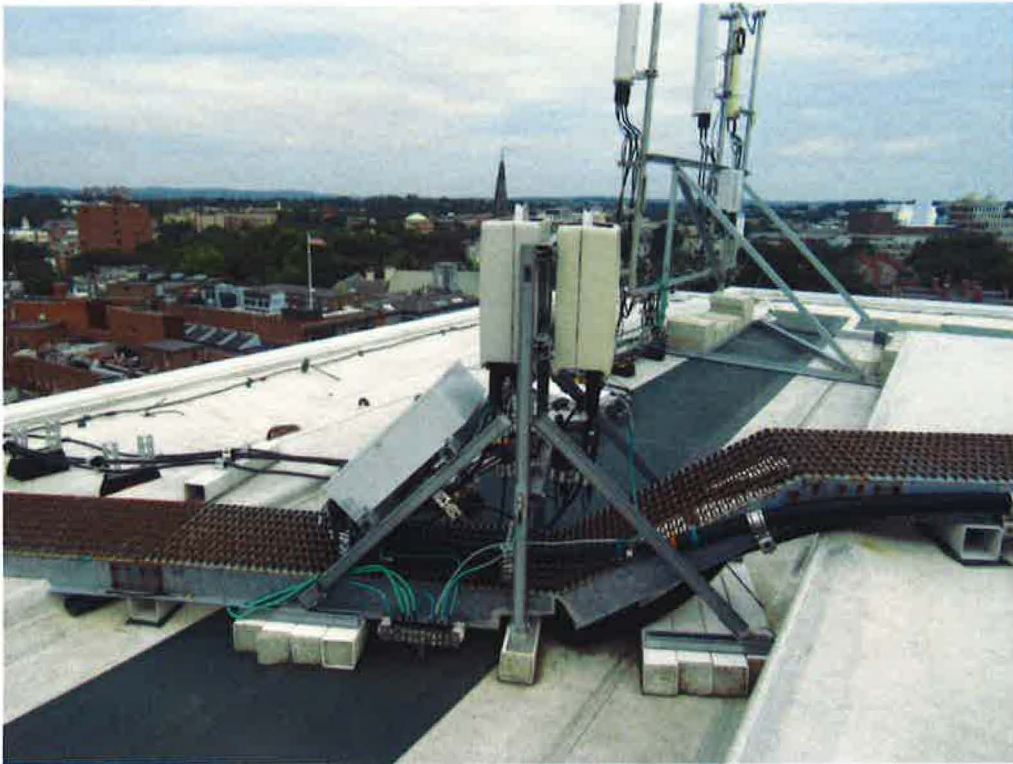
Photo 3: Sample photo illustrating the existing RRH ballast frame.
