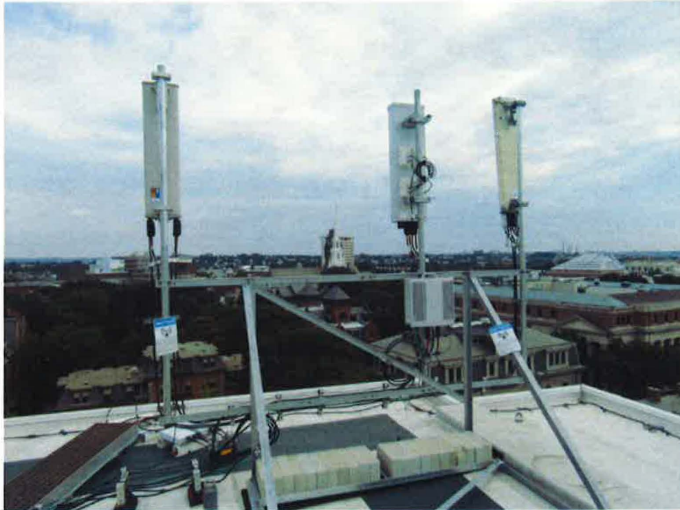
Photo 1: Sample photo illustrating the existing alpha/gamma sector ballast frame.
