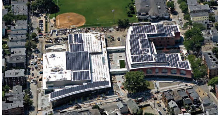
Cambridge is committed to maximizing the amount of renewable energy installed on its schools. The King Open/CSUS and Community Complex will host the largest solar array in the city, with over 4,000 solar panels.
