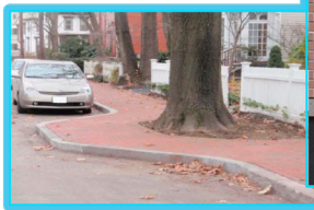
Curb Extensions & Ramps [for accessibility]
