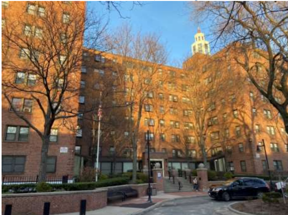
Roosevelt Towers Mid-Rise, off Cambridge Street
