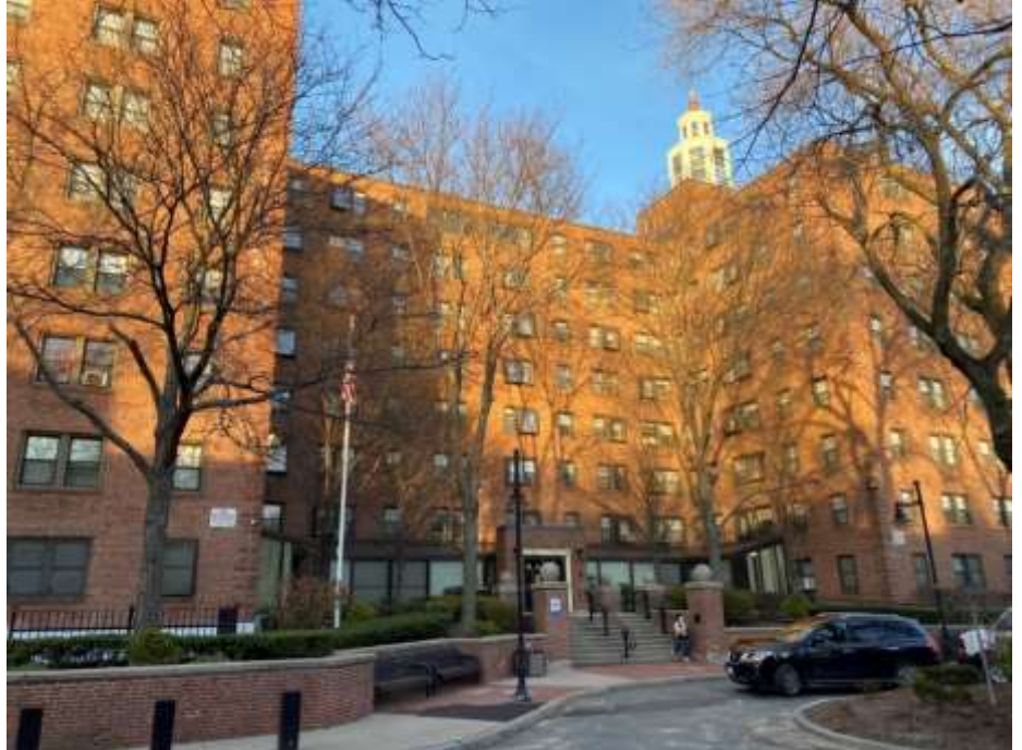
Roosevelt Towers Mid-Rise, off Cambridge Street
