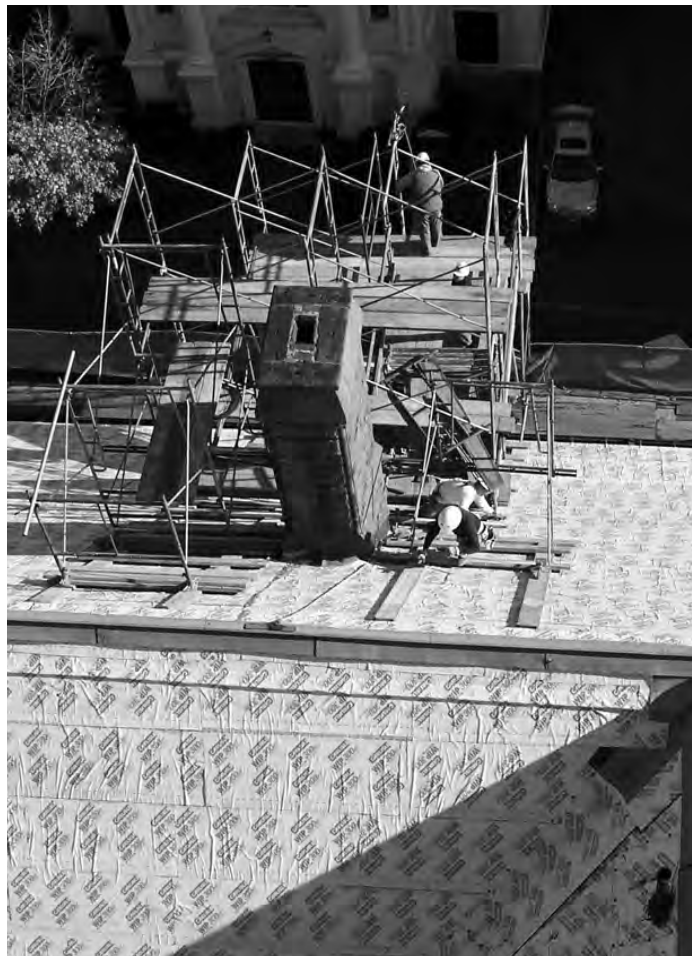
Crews working on the slate roof replacement at City Hall to preserve it as a historical structure.
