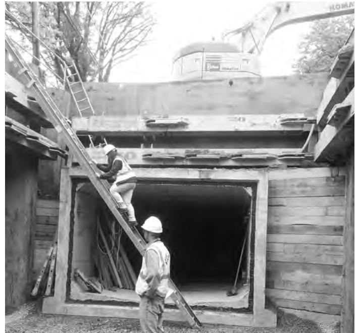
A new 135 foot long stormwater storage tank was constructed on Hovey Avenue. The tank is expected to hold up to 175,000 gallons of water and will alleviate flooding in the mid-Cambridge area.
