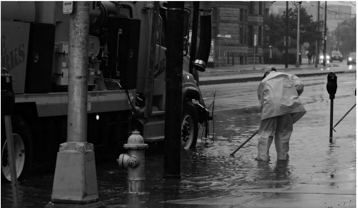
The Sewer Maintenance Division is responsible for over 6,000 catch basins in the city. Here, staff clears a catch basin during Super Storm Sandy in October 2012.
