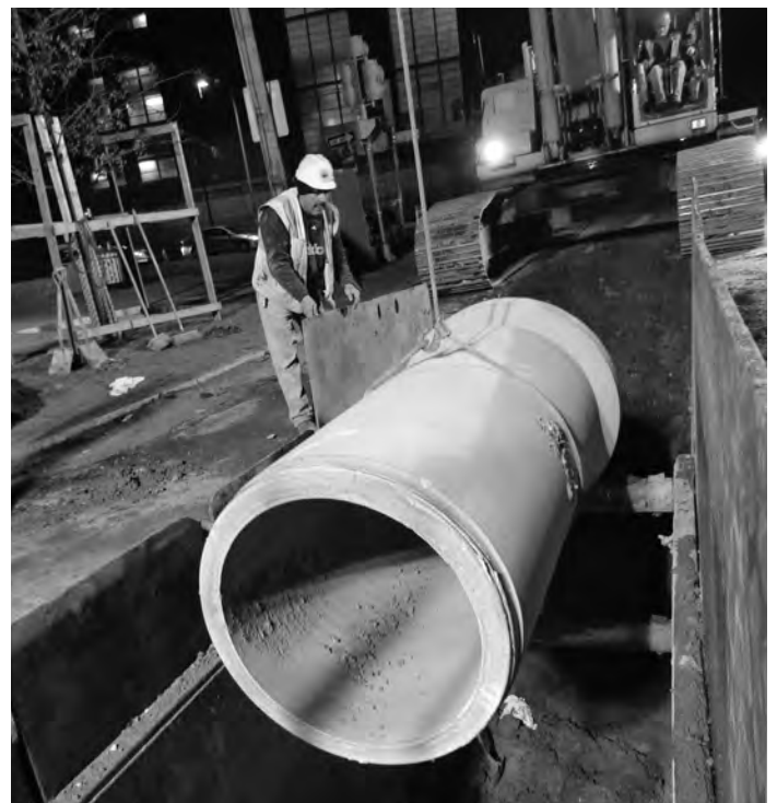
Western Ave construction crews install a 48" drain pipe underneath Memorial Drive that will lead to the new stormwater outfall at the Charles River.
