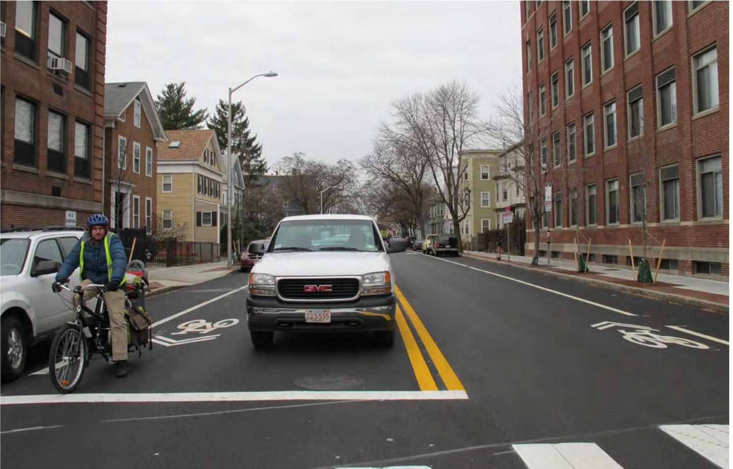
Shared Lane Markings (SLMs) or “sharrows,” are road markings used to indicate a shared lane environment for bicycles and automobiles. Among other benefits, SLMs reinforce the legitimacy of bicycle traffic on the street, recommend proper bicyclist positioning, and may be configured to offer directional and wayfinding guidance.
