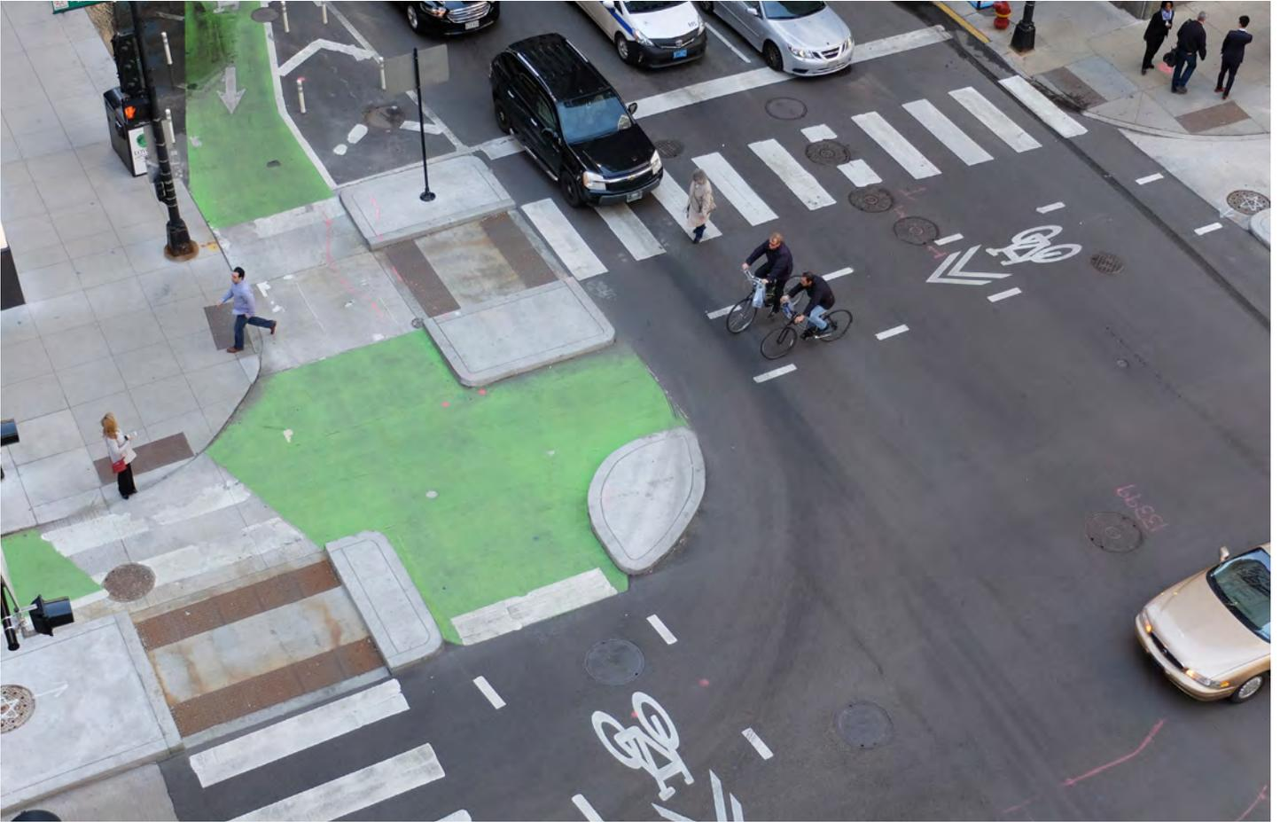
Protected intersections are extensions of existing curblines that provide bicyclists with vertical and horizontal separation from motor vehicles through an intersection. They are typically constructed of concrete, however may also use quick-build materials as interim facilities.
