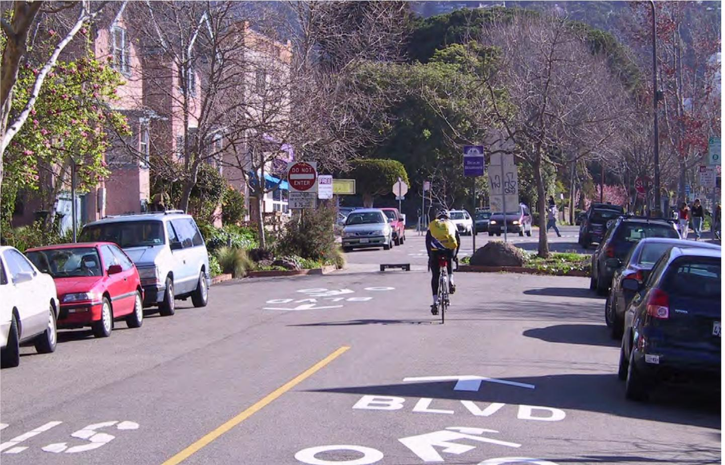
Bike boulevards are streets with low motorized traffic volumes and speeds, designated and designed to give bicycle travel priority. Bike boulevards use signs, pavement markings, and speed and volume management measures to discourage through trips by motor vehicles and create safe, convenient bicycle crossings of busy arterial streets.
