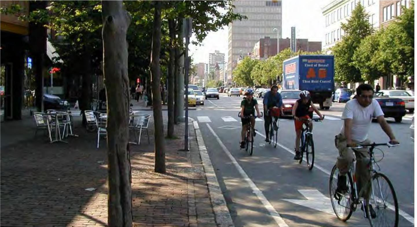
Bike lanes designate an exclusive space for bicyclists through the use of pavement markings and signage. The bike lane is located adjacent to motor vehicle travel lanes and flows in the same direction as motor vehicle traffic. Bike lanes are typically on the right side of the street. Benefits include providing obvious space on the road for cyclists and sending a message to other road users to expect cyclists.
