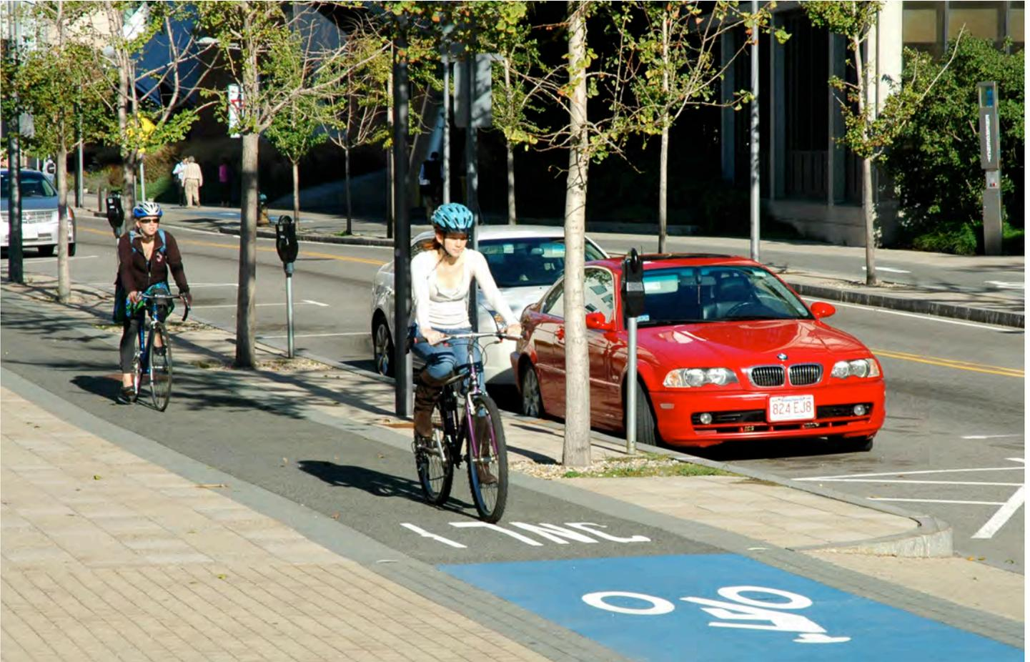
Raised separated bike lanes are bicycle facilities that are vertically separated from motor vehicle traffic. Many are paired with a furnishing zone between the bike lane and motor vehicle travel lane and/or pedestrian area. Benefits include that motorists are kept from easily entering and it is more attractive to a wider range of bicyclists at all levels and ages than less separated facilities.
