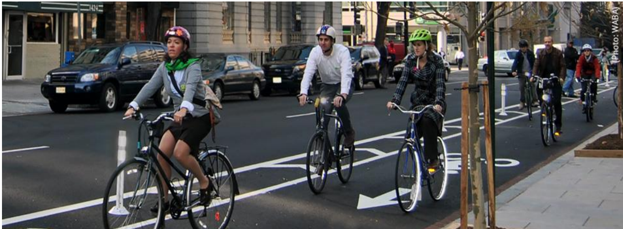
A typical separated bike lane against a curb
