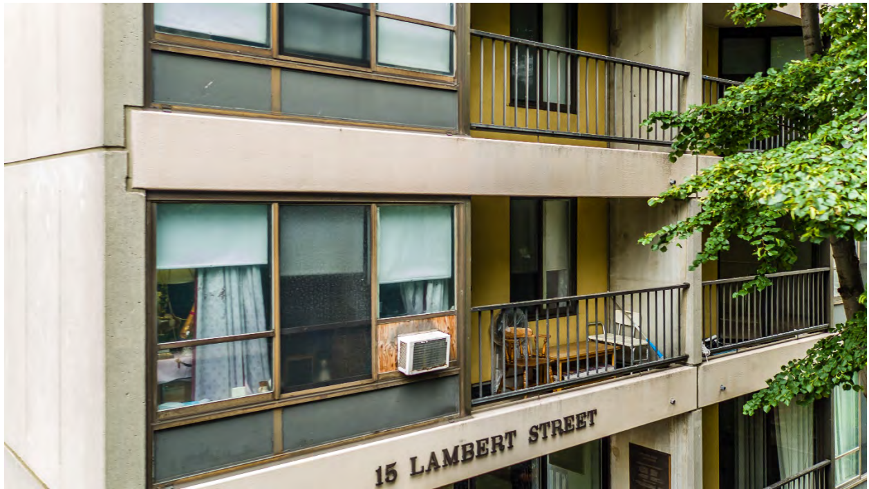
Exterior Condition 2 Lower Unit and Balconies
