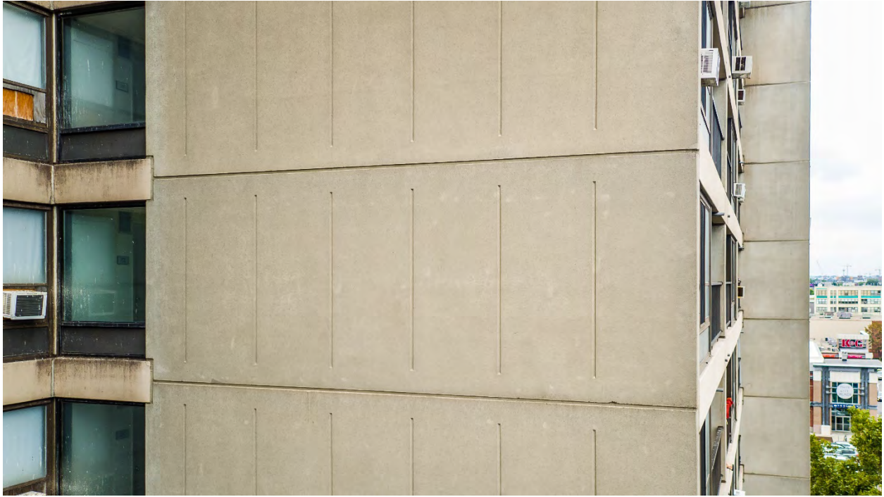
Exterior Condition 1 View along South face
