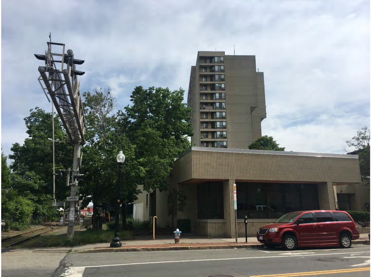
Millers River viewed from South 3 Cambridge Street in Foreground, Community Center and Tower in Background, Railroad tracks to West
