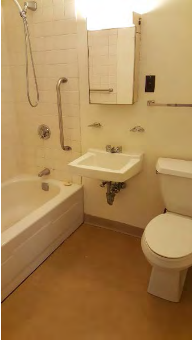
Interior Conditions 5 Typical Unit Bathroom
