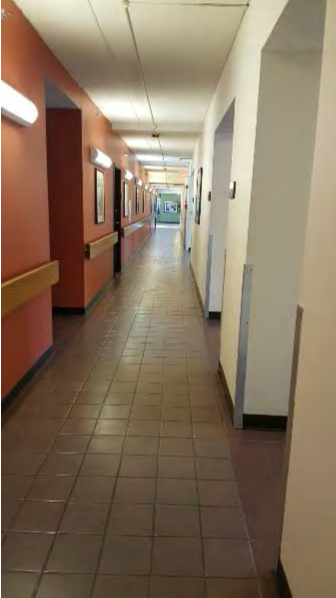
Interior Conditions 3 First Floor Common Area Circulation
