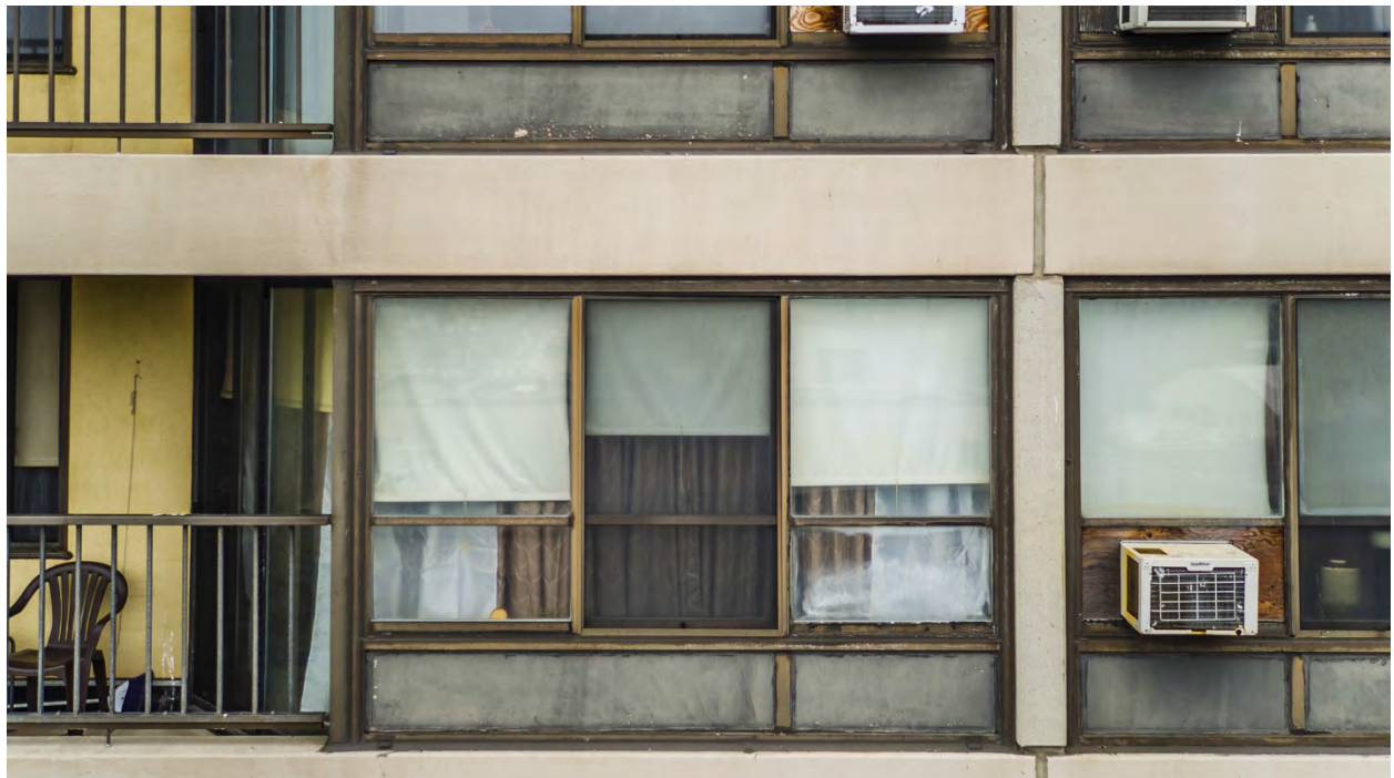
Exterior Condition 3 Upper Units and Balconies
