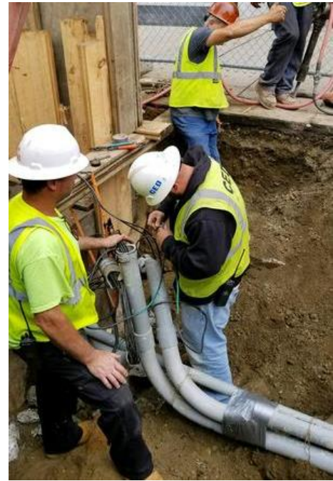
Electrical staff repair an underground conduit.
