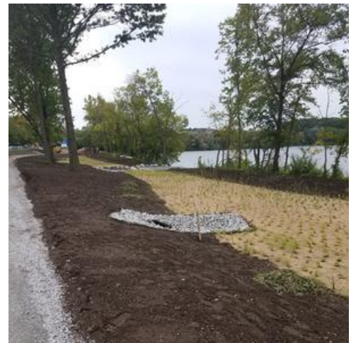
A bio-swale permitted by the Conservation Commission and installed as part of the Fresh Pond Drainage and Community Garden Project.
