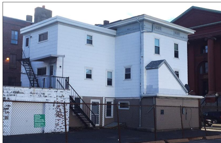
207 Cambridge Street rear and west side. CHC photo, 2016
