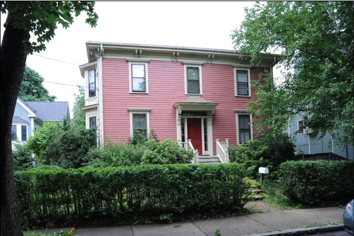
Fig. 7. 27 Cogswell Avenue, 1857. S. L. Willard, builder
