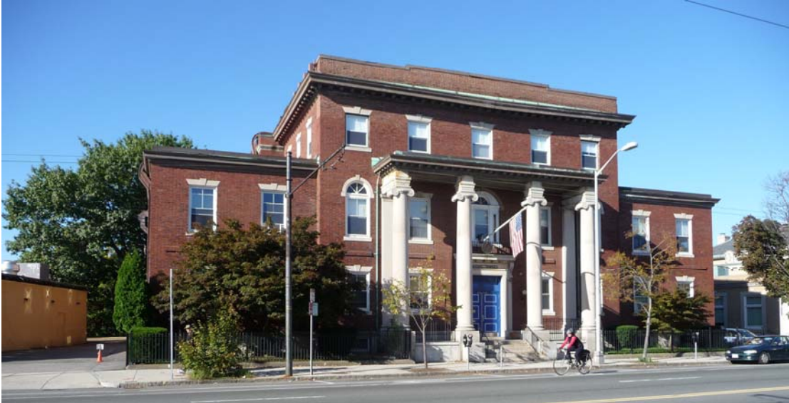
Cambridge Masonic Association building, 1950 Massachusetts Avenue. Photo 2009
