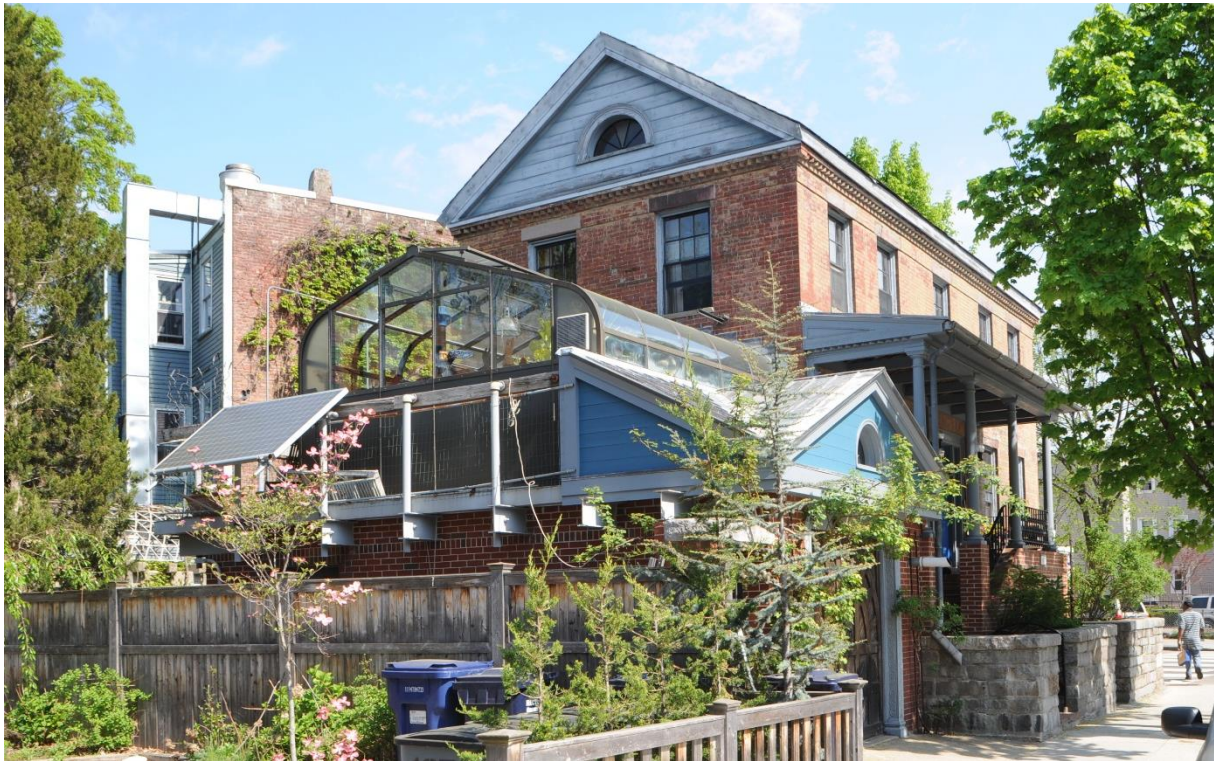
145 Elm Street, showing the garage, greenhouse, solar panel, May 11, 2015
