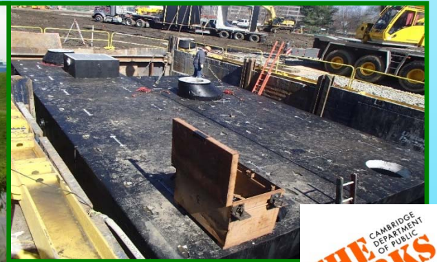
Sewer storage tank
