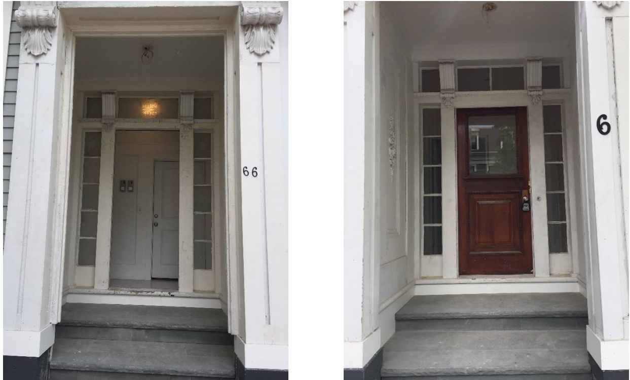
Recessed entries at 66 (left) and 68 (right) June 2017. The trim and etched glass, where existing, has been preserved in place, but a replacement door has not yet been installed at 66. Finish carpentry and paint are incomplete.
