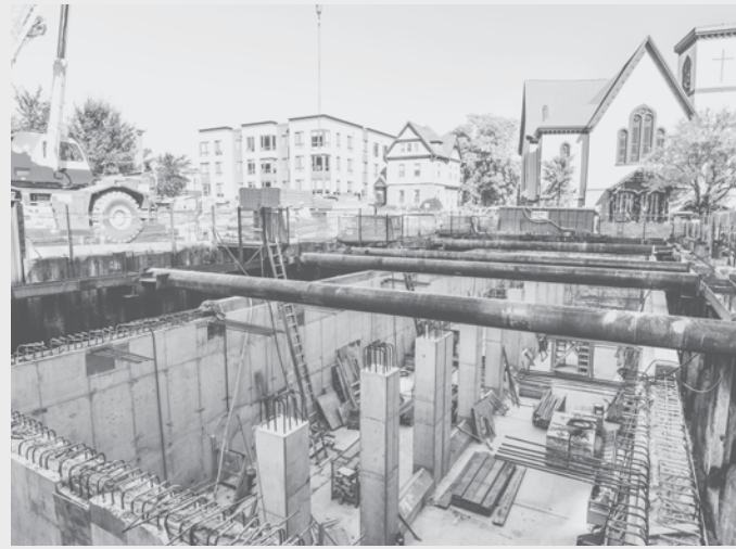
The PL6 tank in The Port
