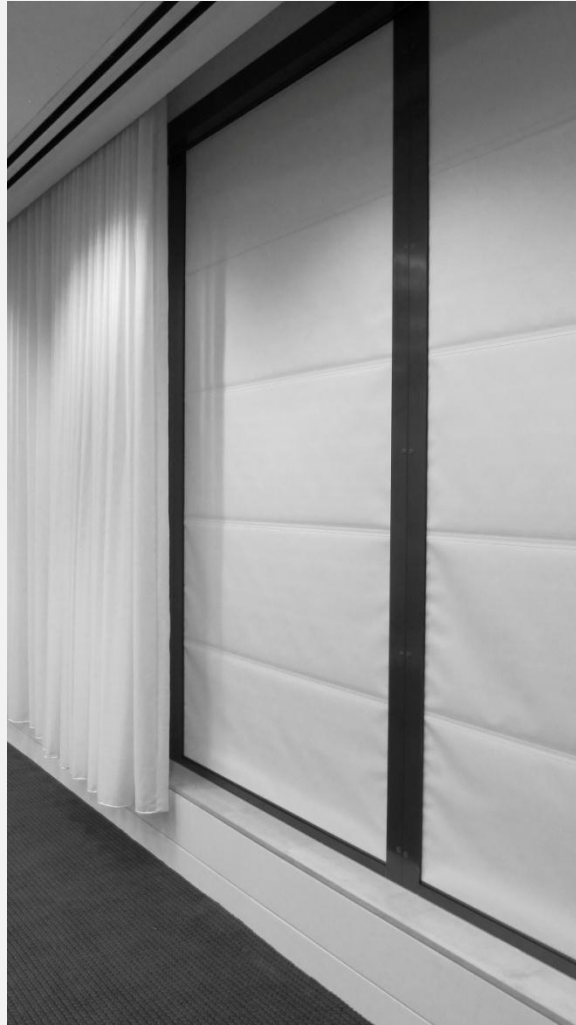
Movable shading with electronic controls - “Provide...glare control devices for all regularly occupied spaces” LEED v4, EQ Credit: Daylight
