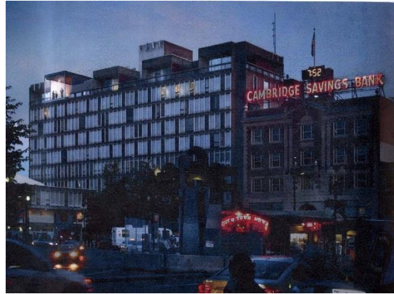
Existing North Holyoke façade from Harvard Yard Initial Design Proposal for Holyoke Facade
