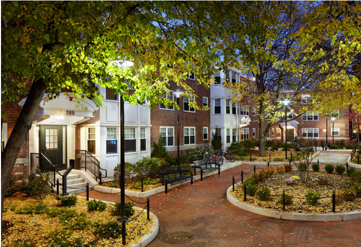
Above: Jackson Gardens, renovation in 2011
