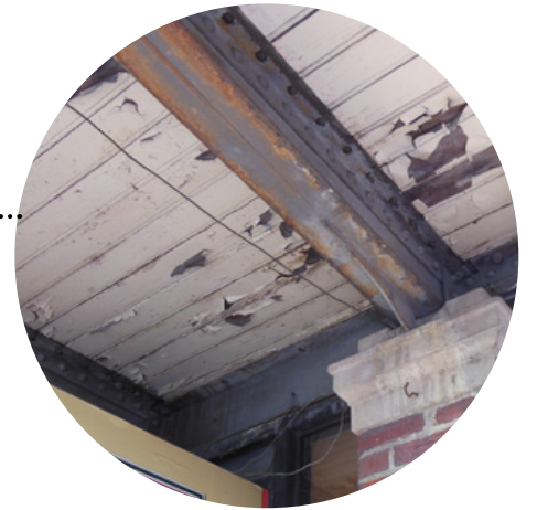
riveted iron structure & exposed wood beadboard
