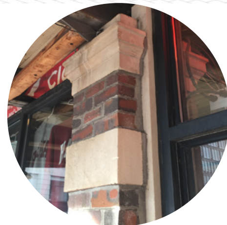
masonry and limestone piers
