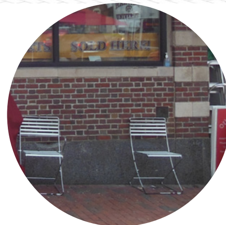
perimeter brick wall with granite base
