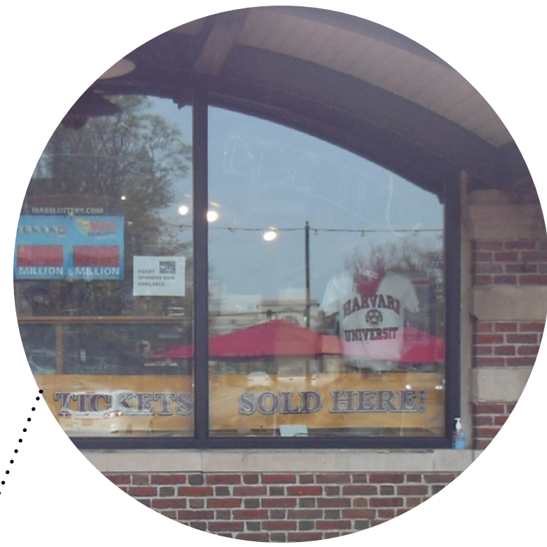
provide new windows
