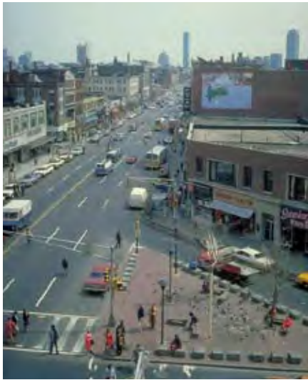
Before improvements were made, Massachusetts Avenue had the character of a highway. Pedestrian crossings were very hazardous and there were no provisions for bicyclists.
