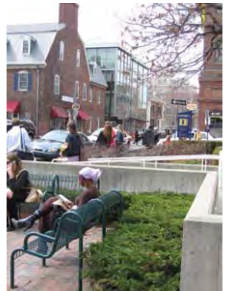
The project at 90 Mt. Auburn was designed to assert its modernity while respecting its historical neighbors.
