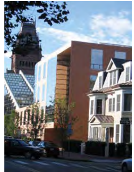
The CGIS building, on the north side of Cambridge Street, is set between an older wood frame structure and the Harvard Graduate School of Design.
