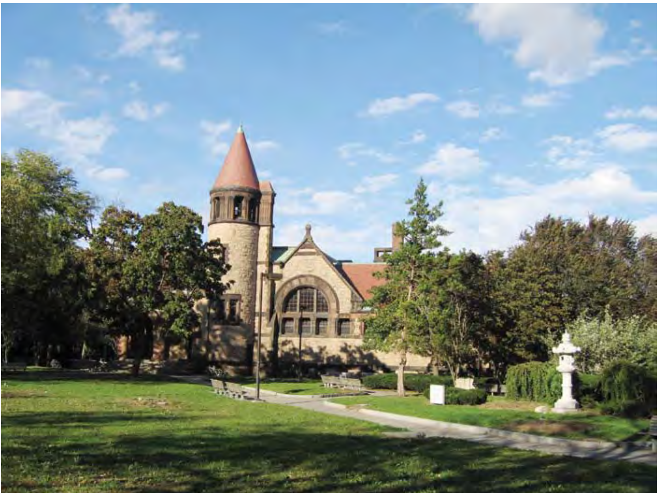
Following a lengthy planning and design process, the Main Library is being thoroughly renovated and will have a glassy new addition.
