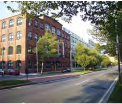
Worthington Place had been a manufacturing facility and warehouse for metal fasteners.
