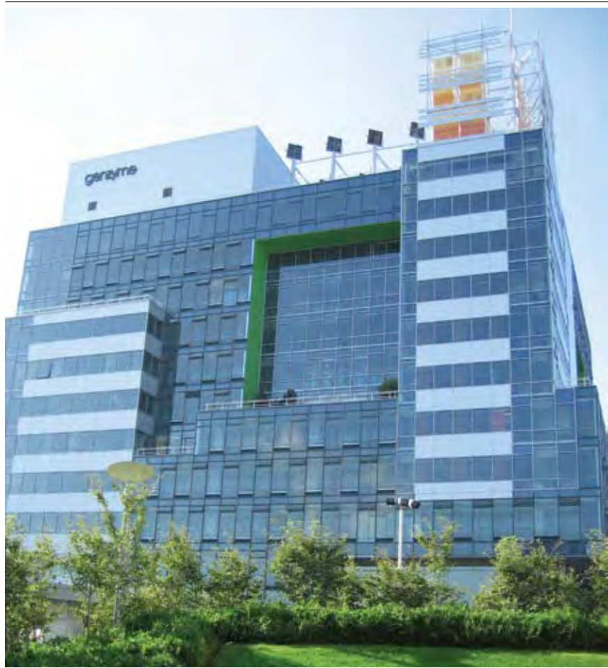
The Genzyme building received a platinum rating from LEED. Its many green features include mirrors on the roof that track the sun to send light down into the beautiful atrium at the heart of the building's interior.
