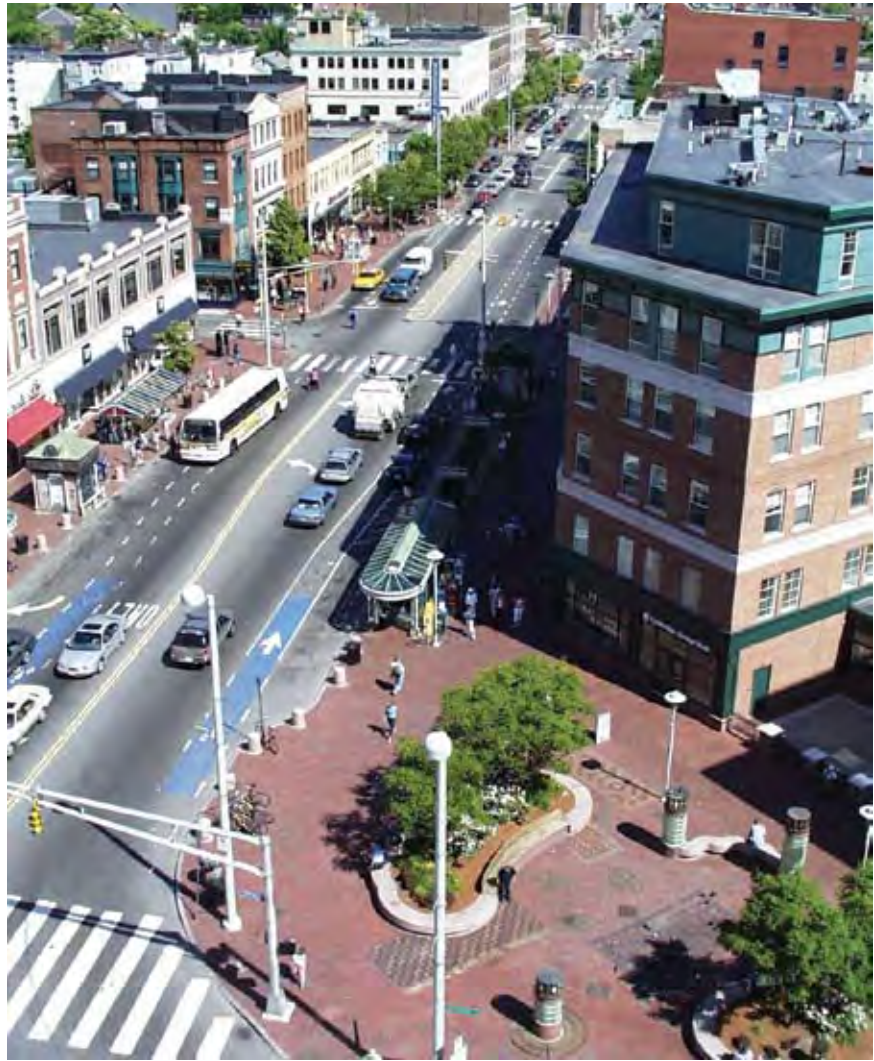
The improved public realm in Central Square, with Carl Barron Plaza in the foreground. Sidewalks were widened and pedestrian crossings were clearly delineated. Bicycle lanes were provided.
