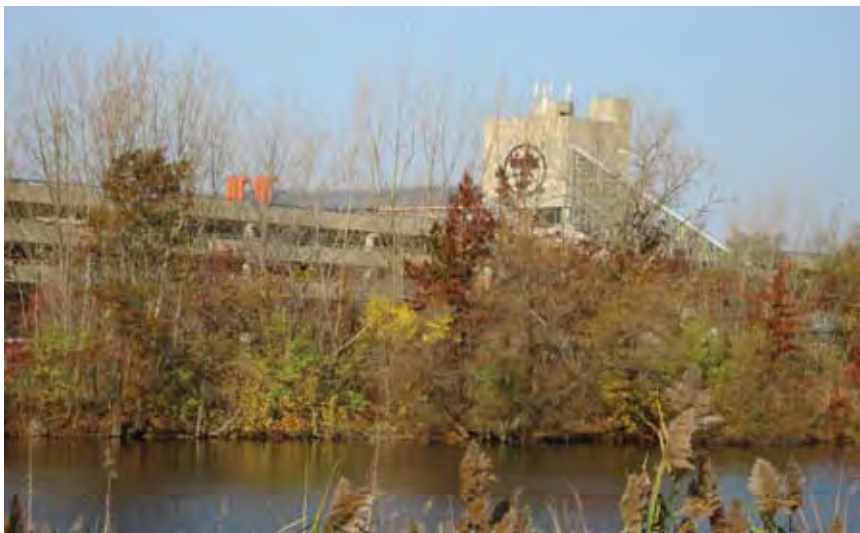
Alewife, with its extensive wetlands, includes a mix of business, retail, and residential uses near the transit station at the terminus of the Red Line.
