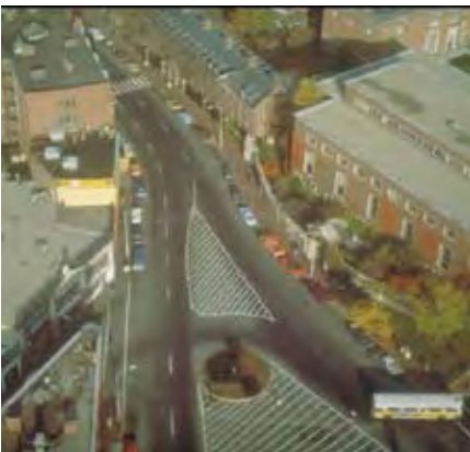
Quincy Square was an unattractive and hazardous intersection. It was unclear how pedestrians should circulate in this sea of asphalt.
