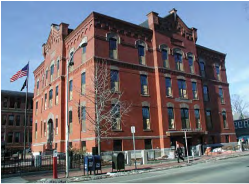
The City Hall Annex has been renovated to LEED standards.
