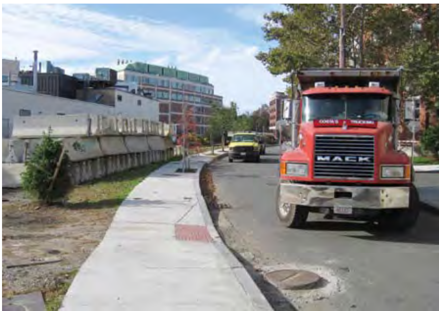
Finishing the streets and sidewalks in the Cambridgeport Roadways Project.
