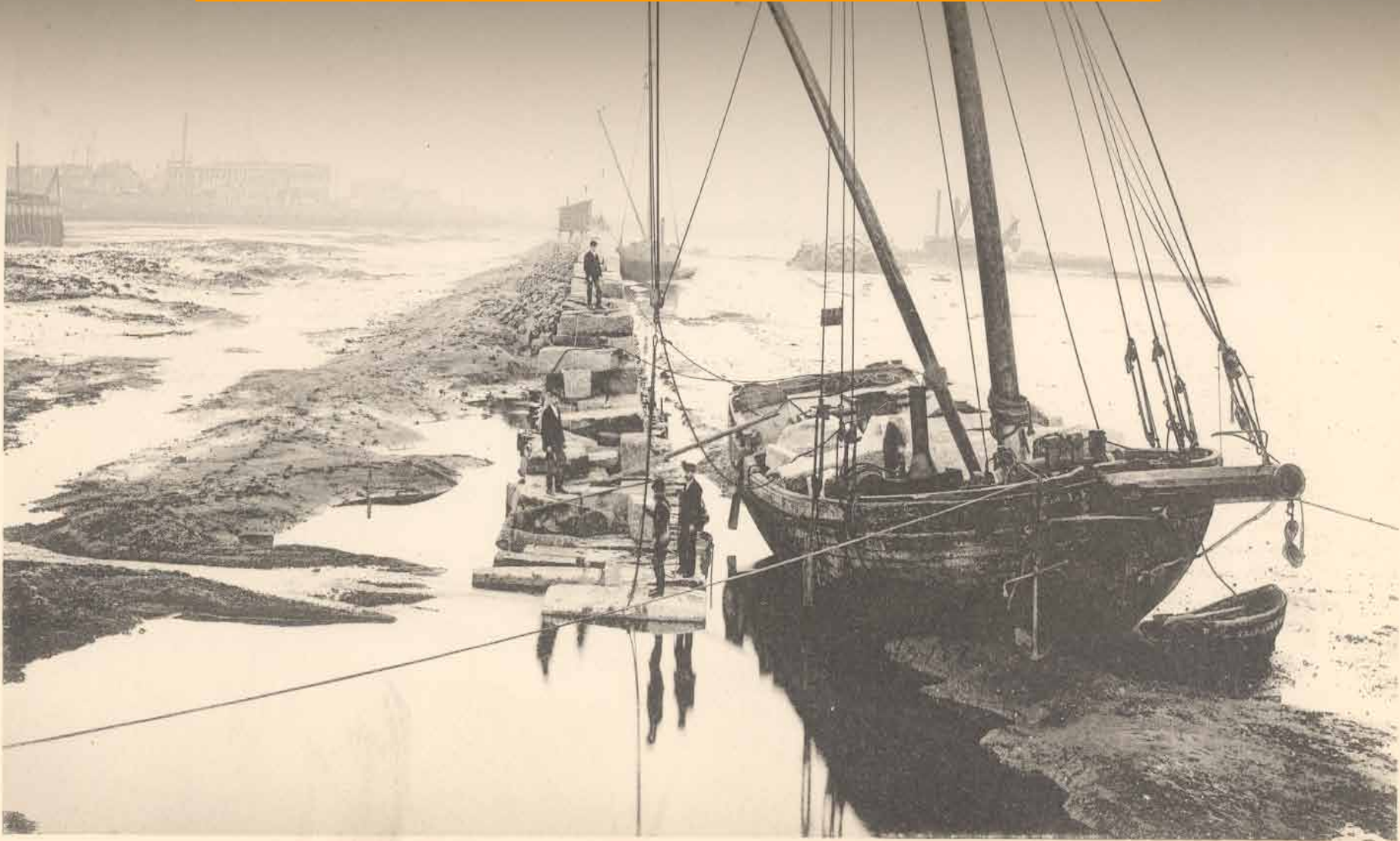
SEA-WALL ON CHARLES RIVER. LOOKING EAST TOWARD MAIN ST.
