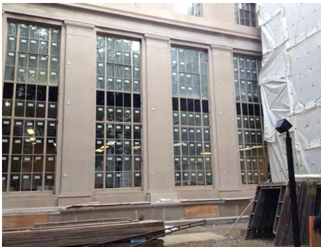
Windows installed as part of Building 2 renovation
