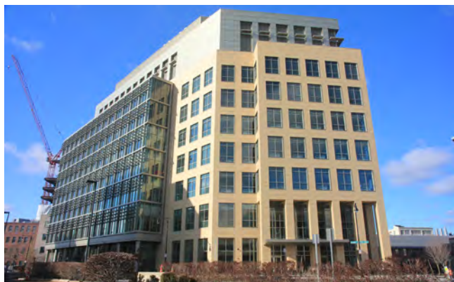
610 Main Street under construction
