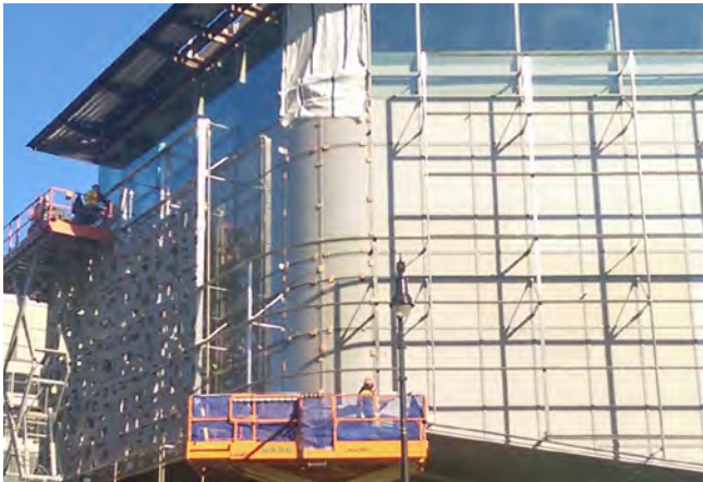
Stone facade construction at 181 Massachusetts Avenue
