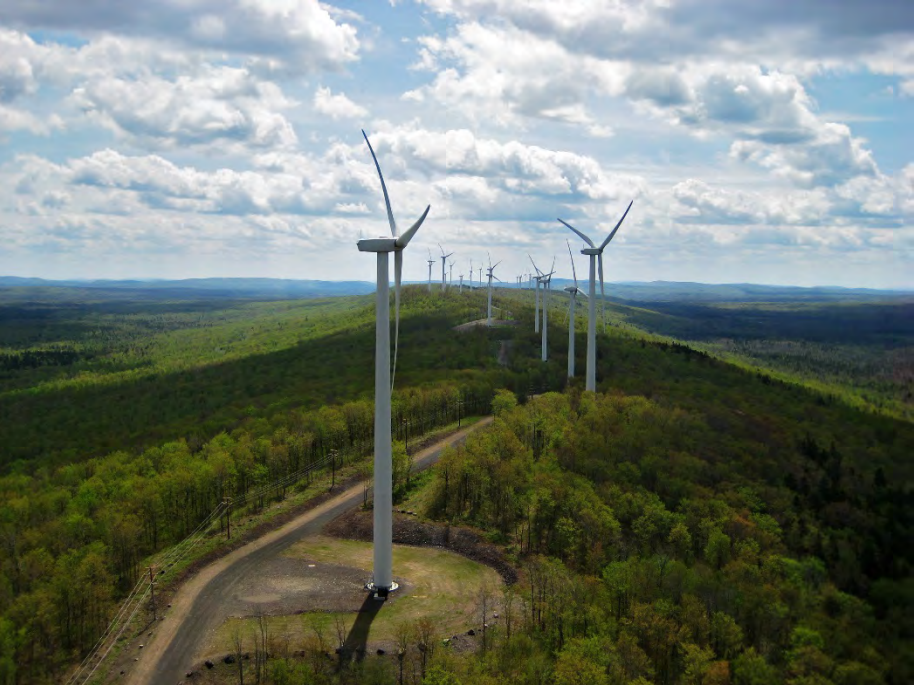
12MW Maine Stetson II wind power PPA (2009)
