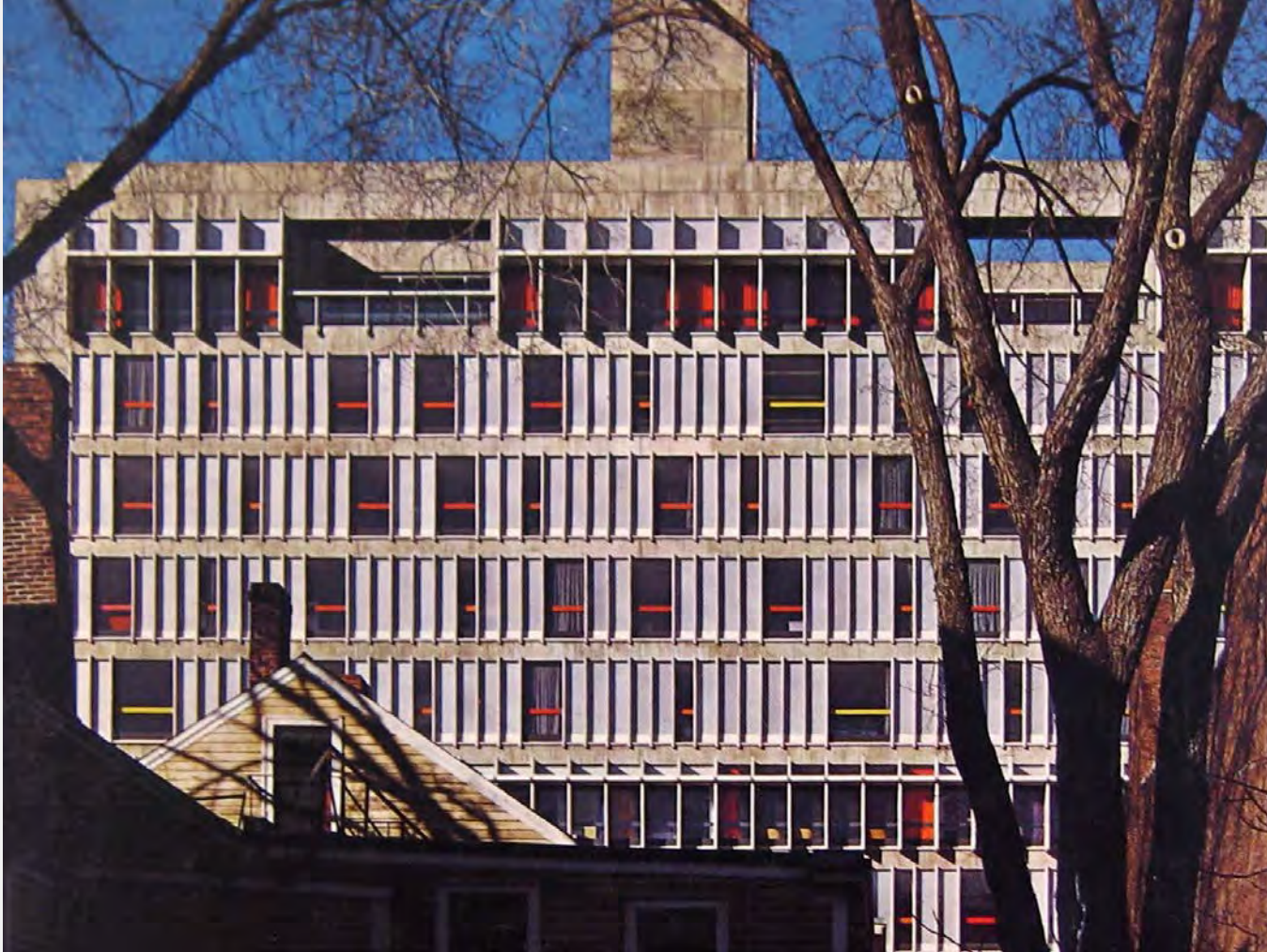
Building facade restoration • Bruner/Cott
