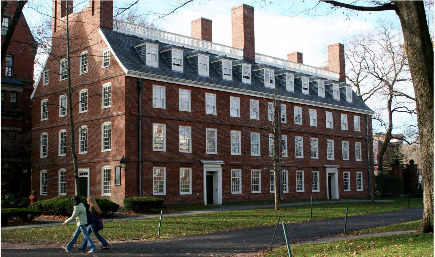
Exterior restoration, HVAC and building systems upgrades | Baker/Wohl Architects
