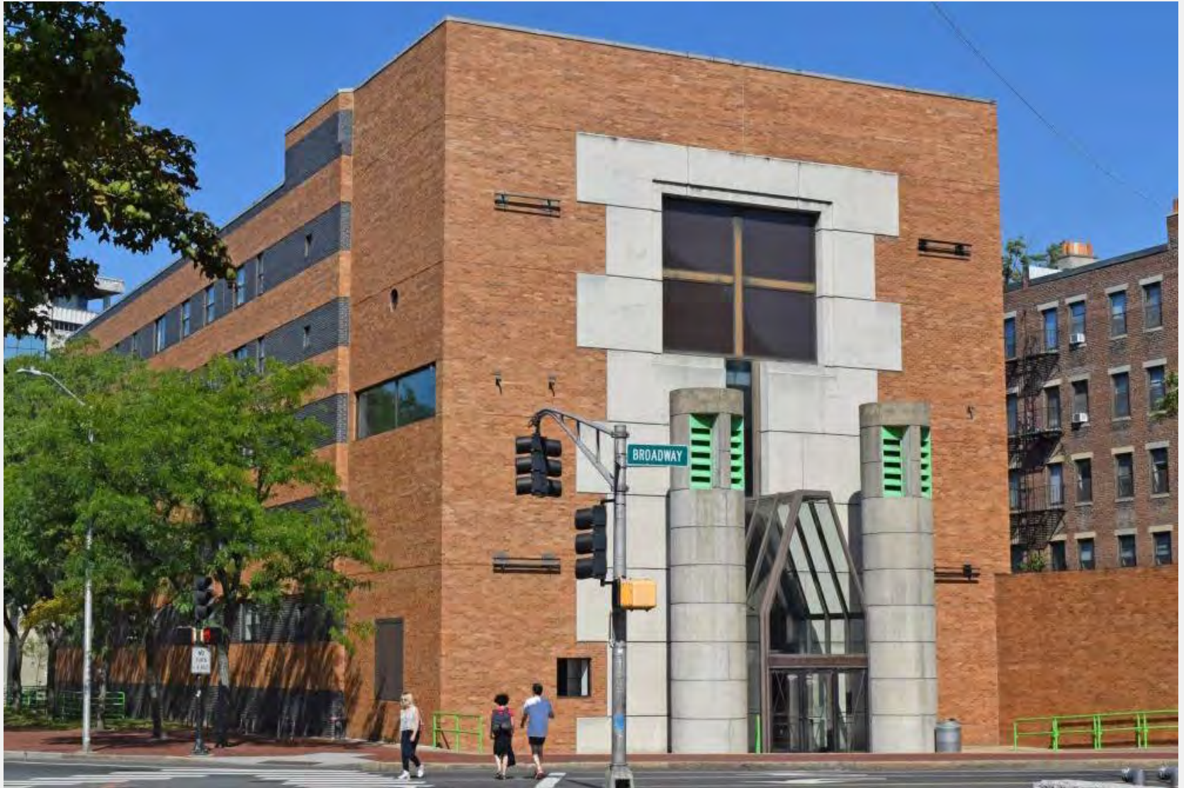
Renew building systems and accommodate new uses | designLAB
