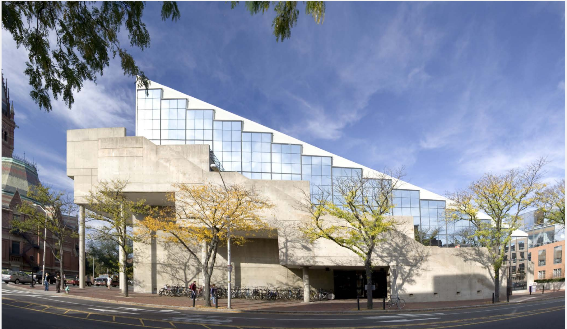
Renovation of teaching facilities | TBD
