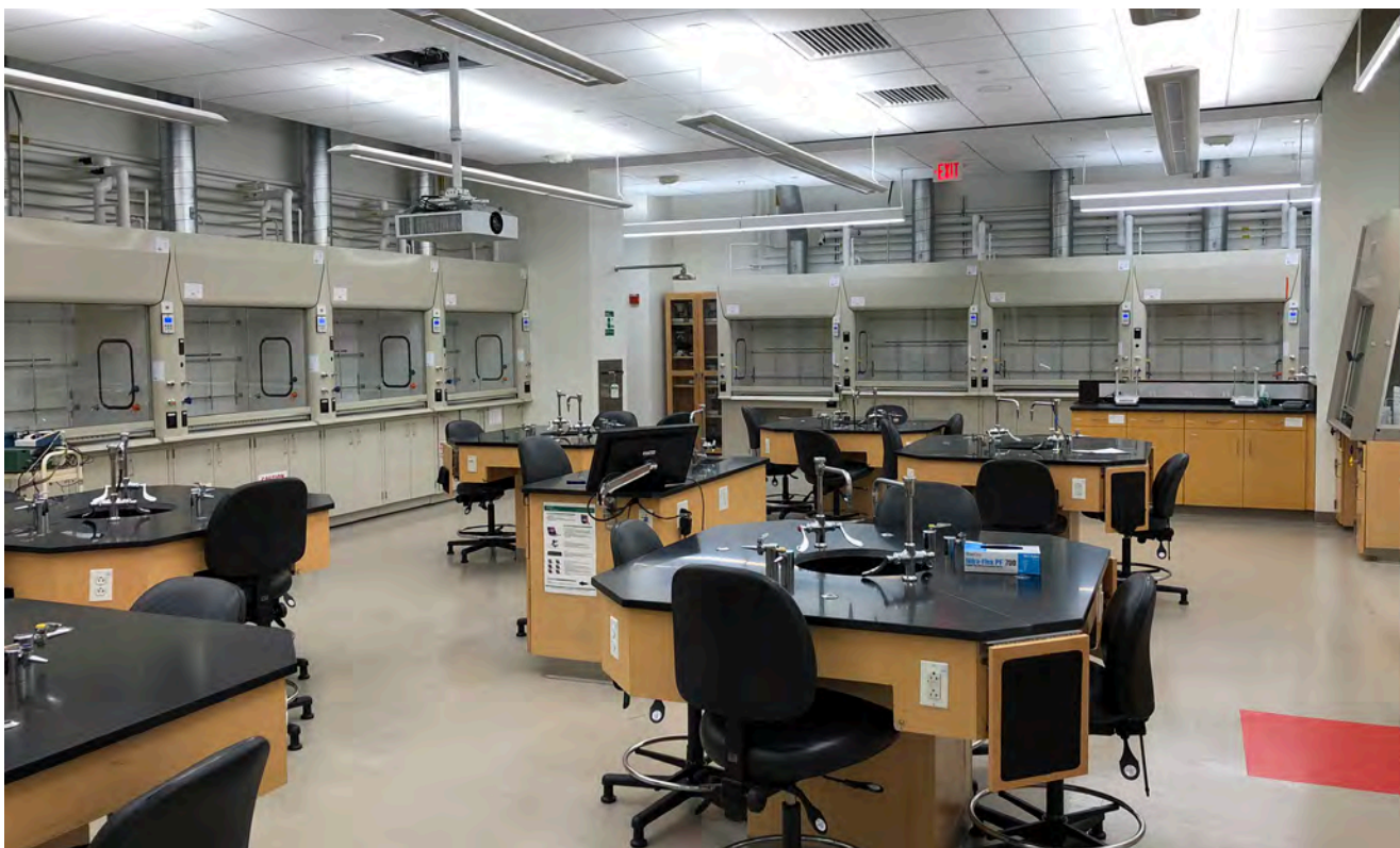
EIGHT NEW (AND ONE EXISTING) FUME HOODS INCREASE CHEMISTRY AND BIOLOGY INSTRUCTION IN THE RENOVATED SCIENCE LAB.
