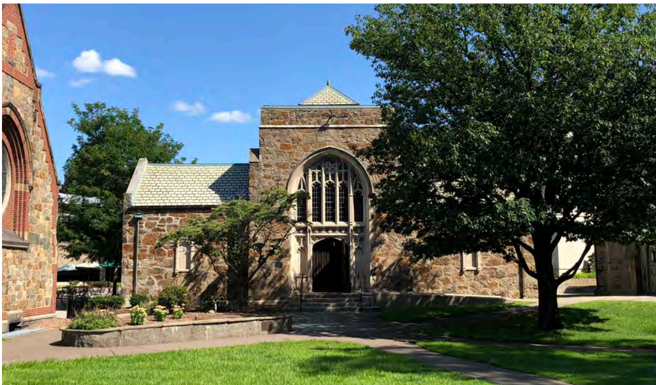
MINOR RENOVATIONS TO WRIGHT HALL WERE COMPLETED THIS SUMMER TO FACILITATE RELOCATION OF THE DEAN'S OFFICE FOR THE COLLEGE OF LIBERAL ARTS AND SCIENCES AS WELL AS THE CONSOLIDATION OF THE BUSINESS DEPARTMENT.
