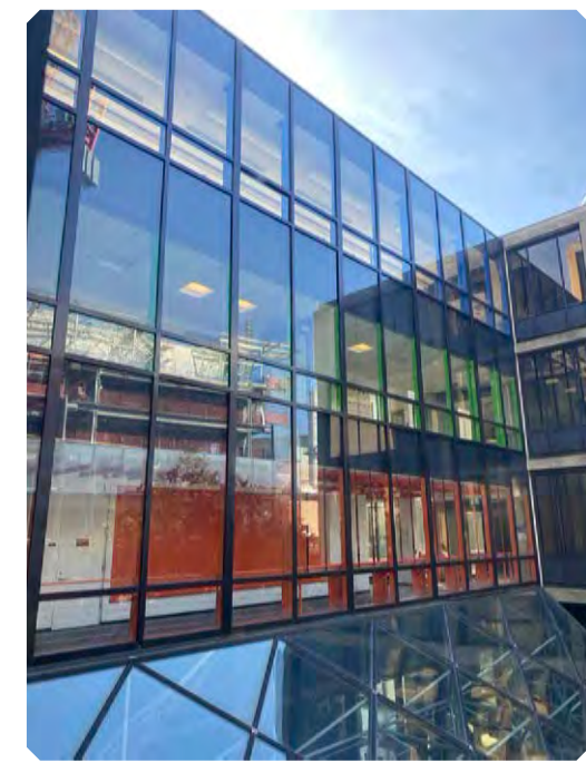
Building 34 Curtain Wall renewal. Image courtesy of MIT Department of Facilities.
