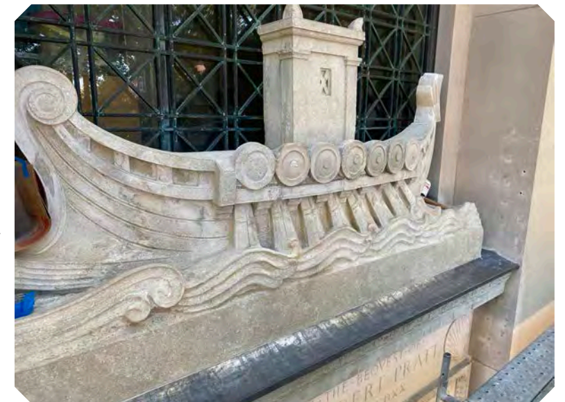
Building 5 ship relief renewal. Image courtesy of MIT Department of Facilities.
