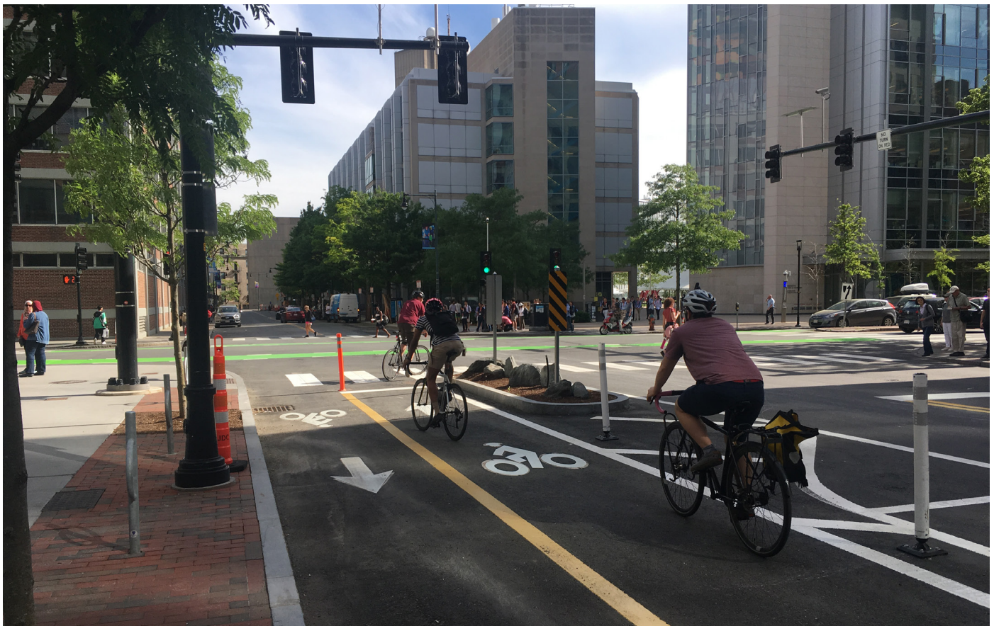
This two-way separated bike lane on Ames Street uses traditional construction and quick-build materials.
