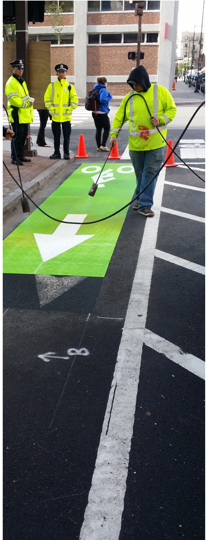
Crew installing bicycle decal and green pavement markings.
