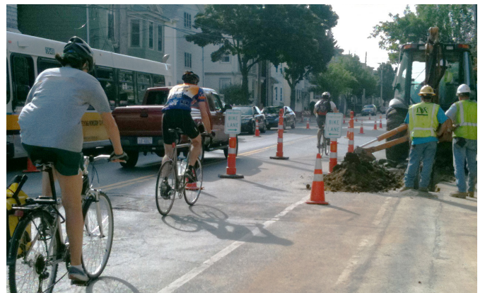
Construction zone featuring temporary bike lane.
