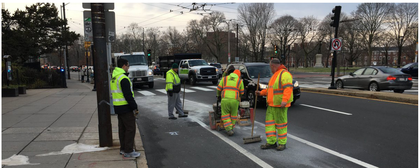
Crew working on bike lanes on Massachusetts Avenue.
