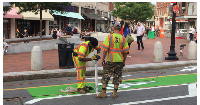
Installation of a new flex post on a separated bike lane.
