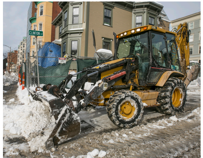
The City uses a variety of tools to clear snow from streets and separated bike lanes.
