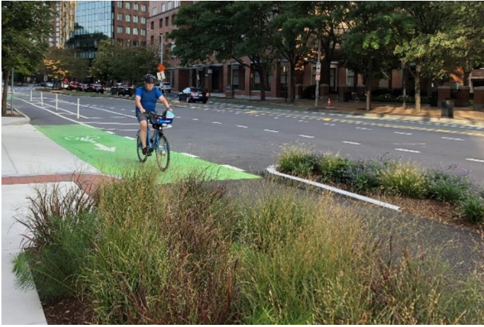
Examples of Separated Bike Lanes in Cambridge. Broadway (left) features a one-way bike lane separated by a planted curb. Brattle Street (right) features a two-way bike lane separated by flex posts and vehicle parking.
