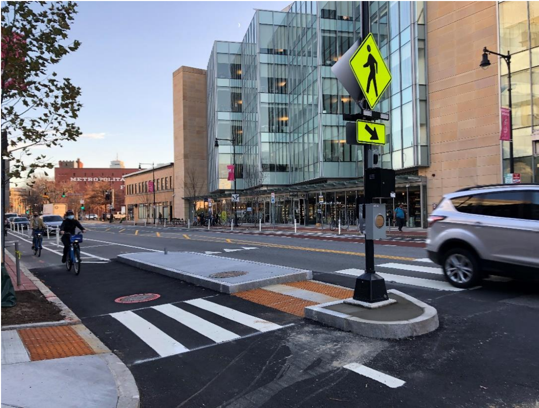
People riding bikes in the separated bike lane that was installed as part of the South Mass. Ave. project; the image also shows the pedestrian island and rapid flash beacon (RRFB) installed to improve the crossing.
