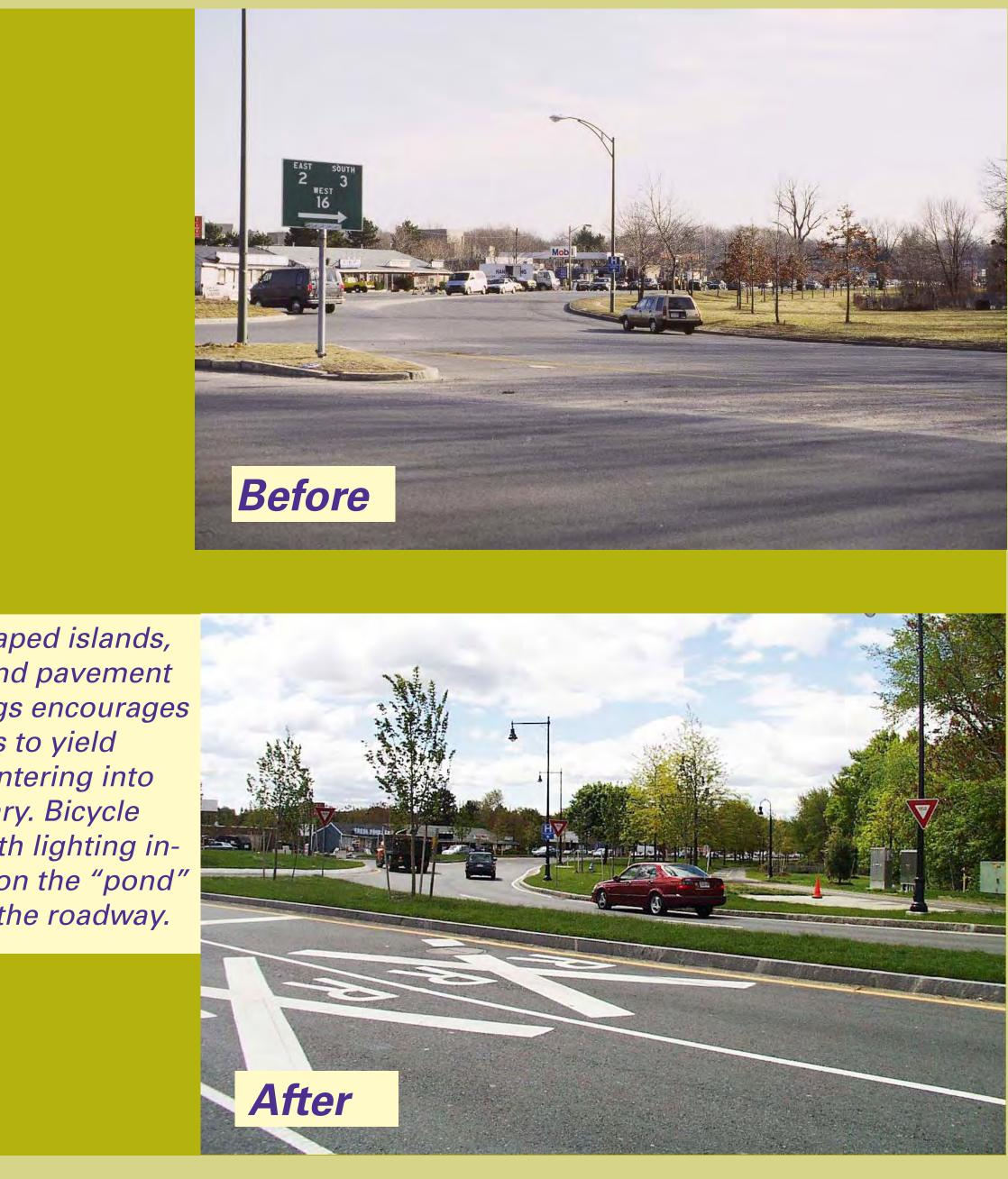
Landscaped islands, signs and pavement markings encourages vehicles to yield when entering into the rotary. Bicycle path with lighting installed on the "pond" side of the roadway.
