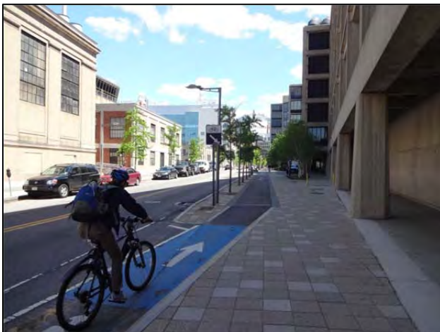
Figure 3: Typical Transition between Facilities on Vassar Street
