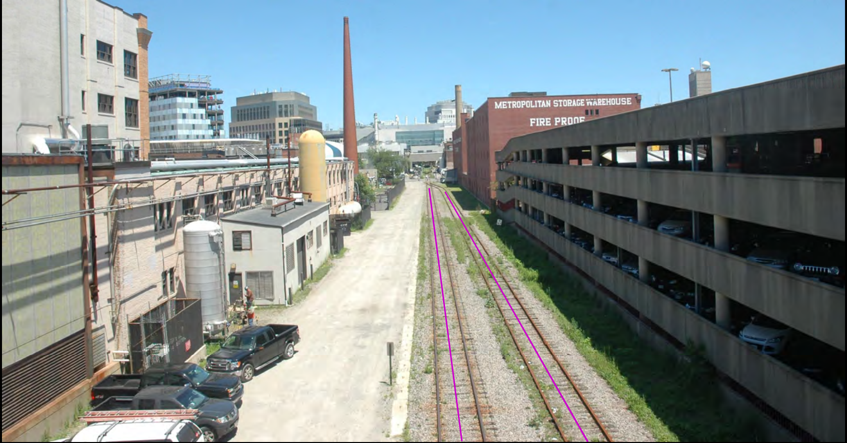
The centerline of the tracks are 13 feet apart.
