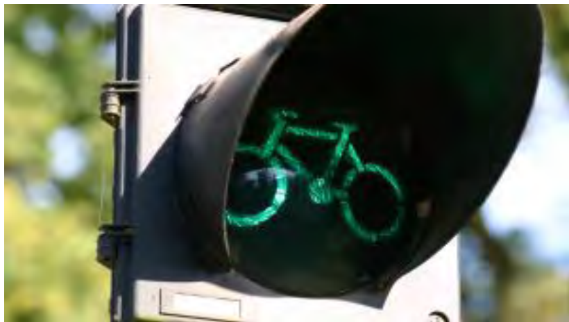
Bicycle Traffic Signal
