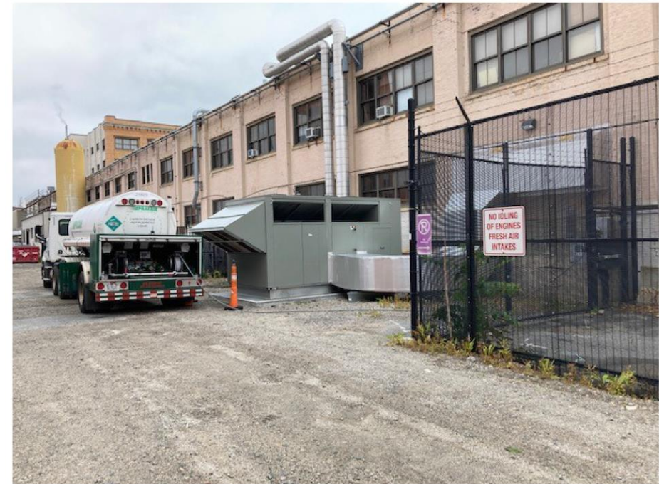
MIT Building Number NW12 Carbon Dioxide delivery photo
