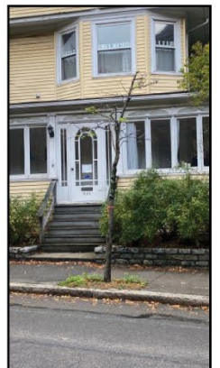
2 248 River St 3.5" cal. Hackberry Poor Condition
