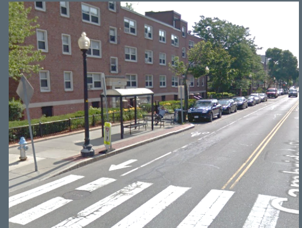
Example of curb extension with bus shelter on Cambridge Street
