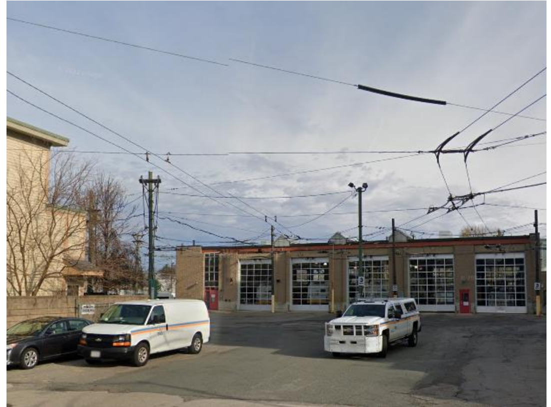
Bus Facility Entrance – Massachusetts Ave
