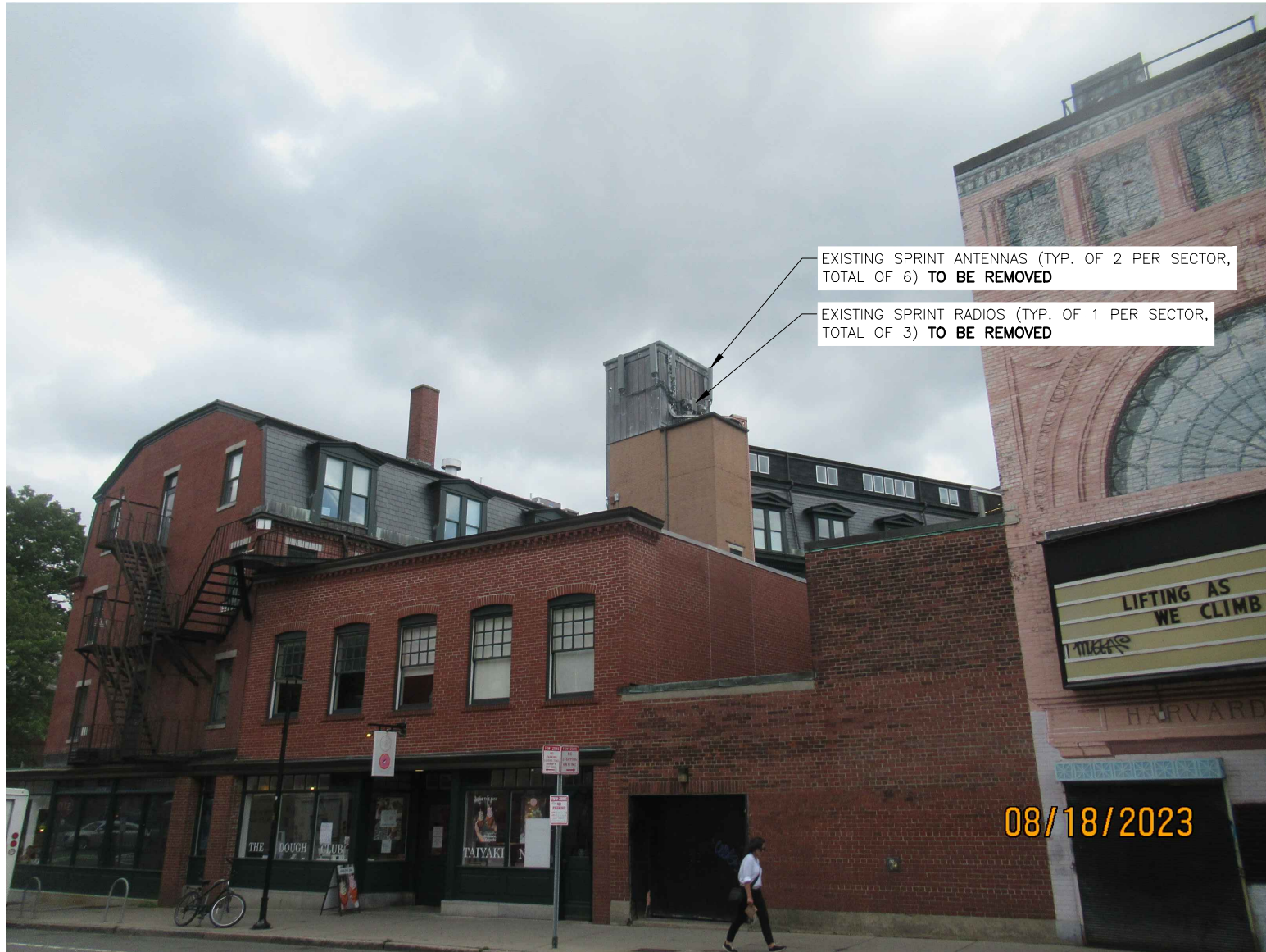
VIEW SOUTHEAST FROM CHURCH ST
