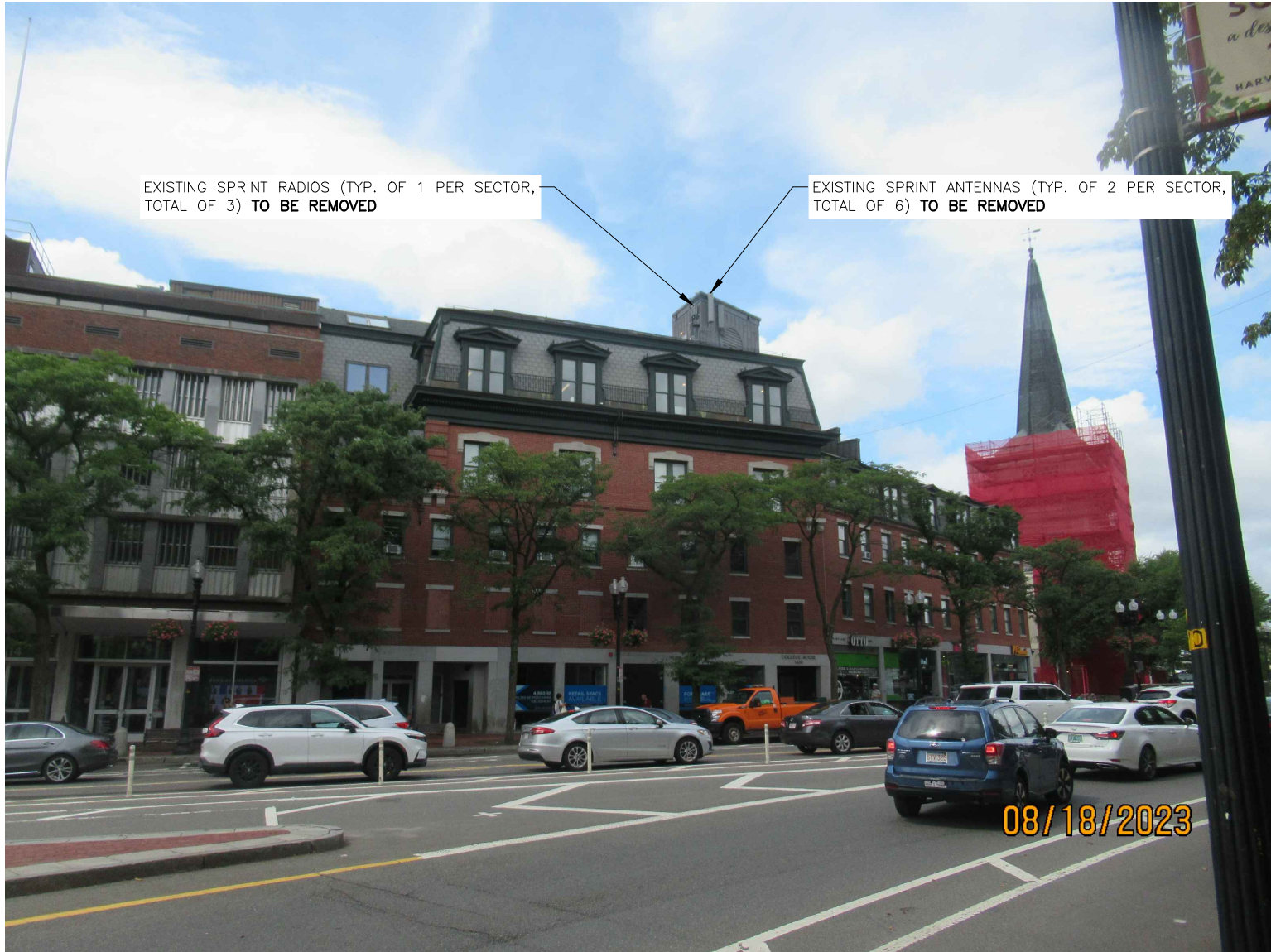
VIEW NORTHWEST FROM MASSACHUSETTS AVE
