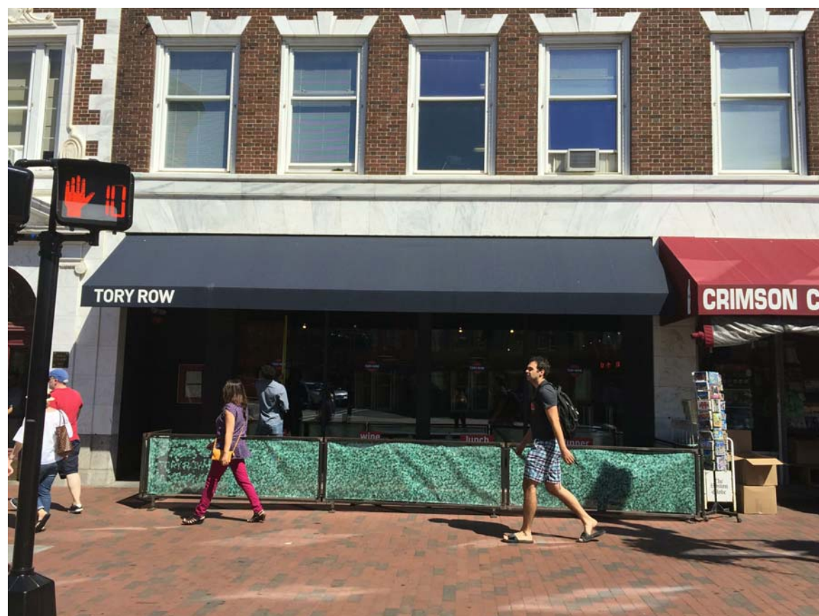
EXISTING TORY ROW FACADE AND PATIO CONDITIONS
