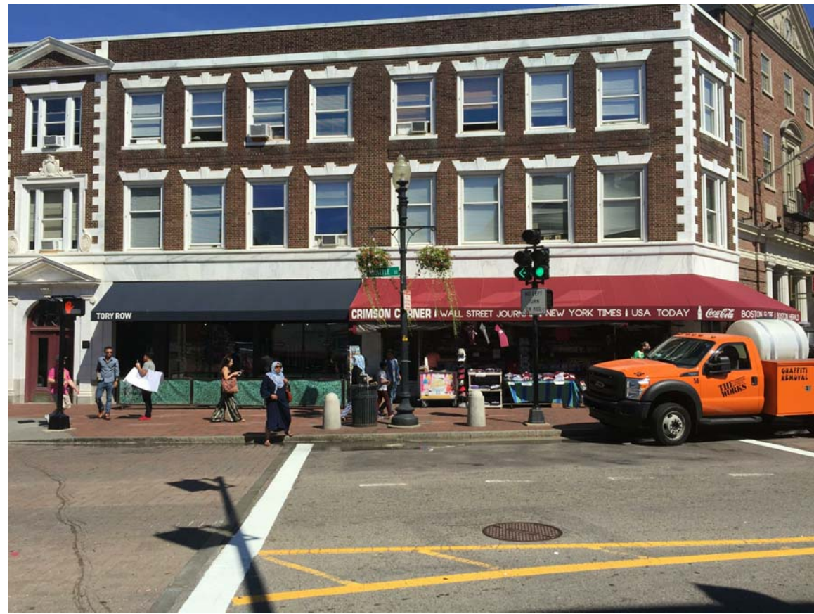
EXTERIOR FACADE AND STREET CONDITIONS. BRICK AND MARBLE TO REMAIN AS IS
