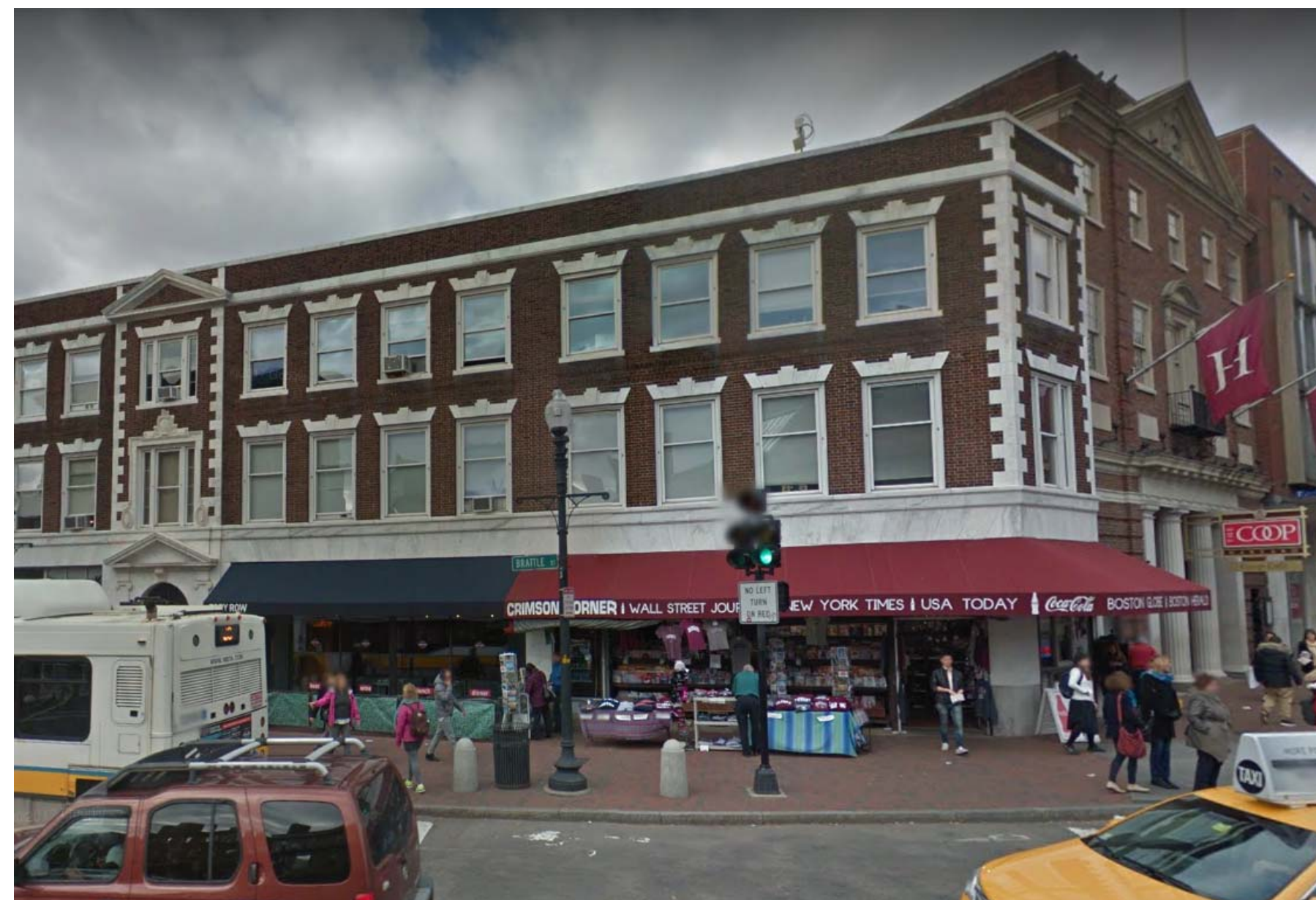
EXISTING EXTERIOR FACADE
