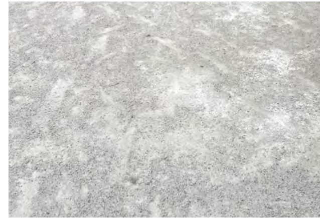
Decomposed Granite Pavement
