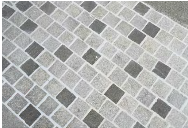
Stone Setts Pavement
