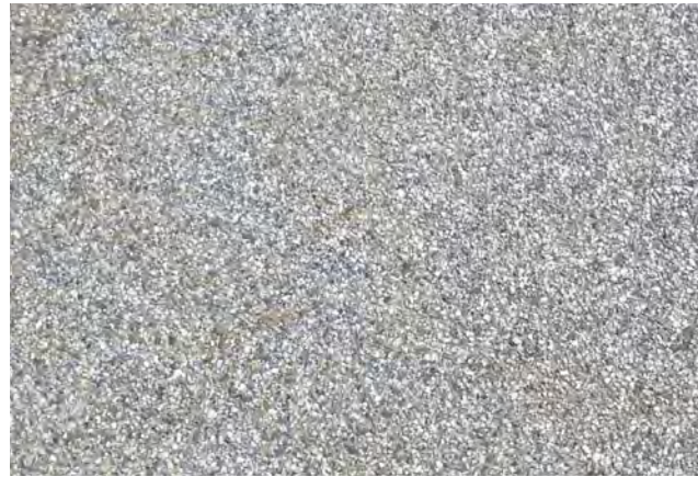
Exposed Aggregate Concrete Pavement
