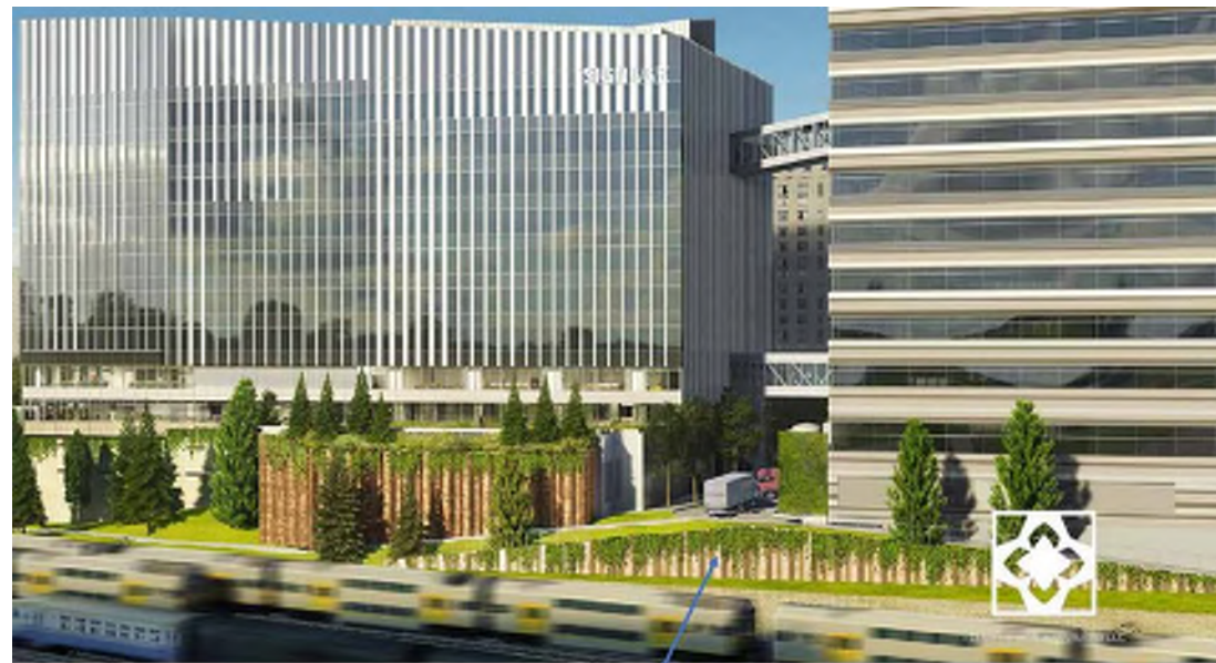
Elevation Change at the North Area of Project Site
