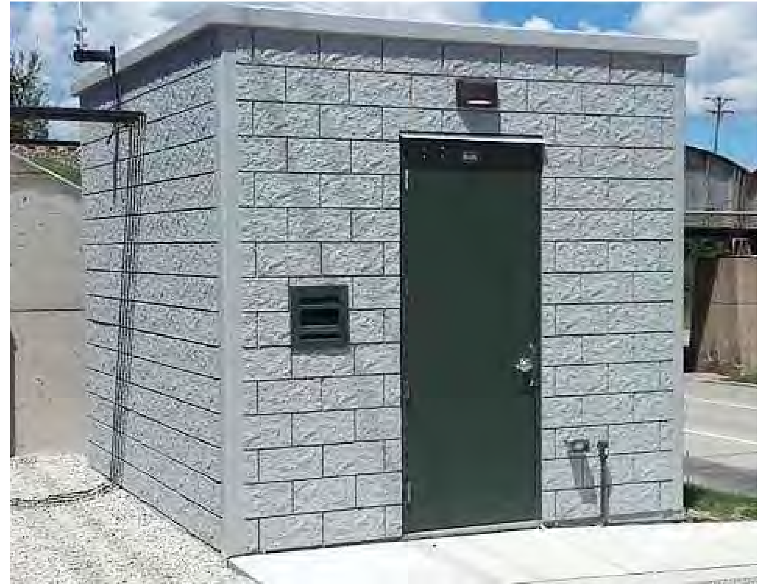
Pump Station Control Building
