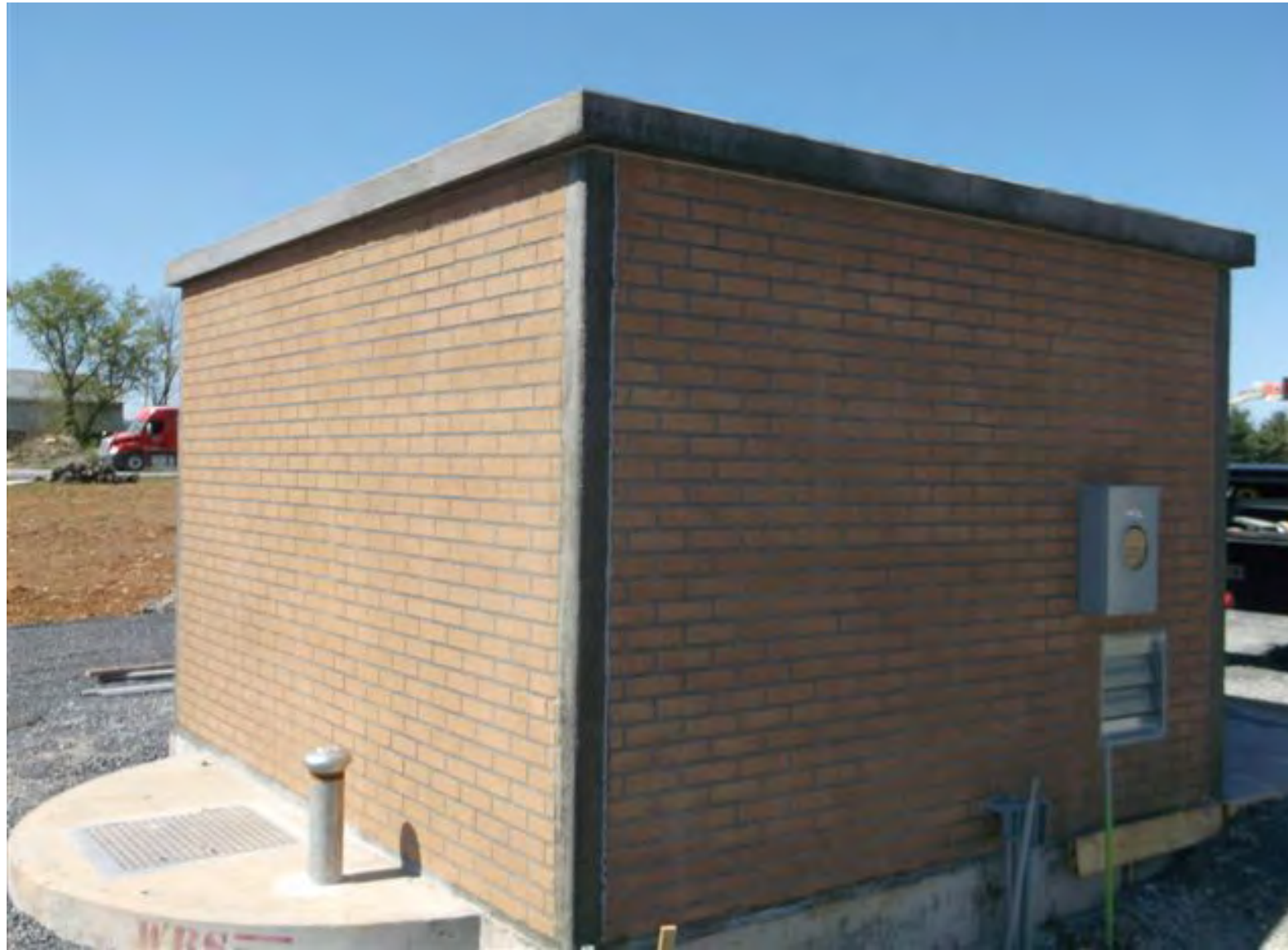
Pump Station Control Building
