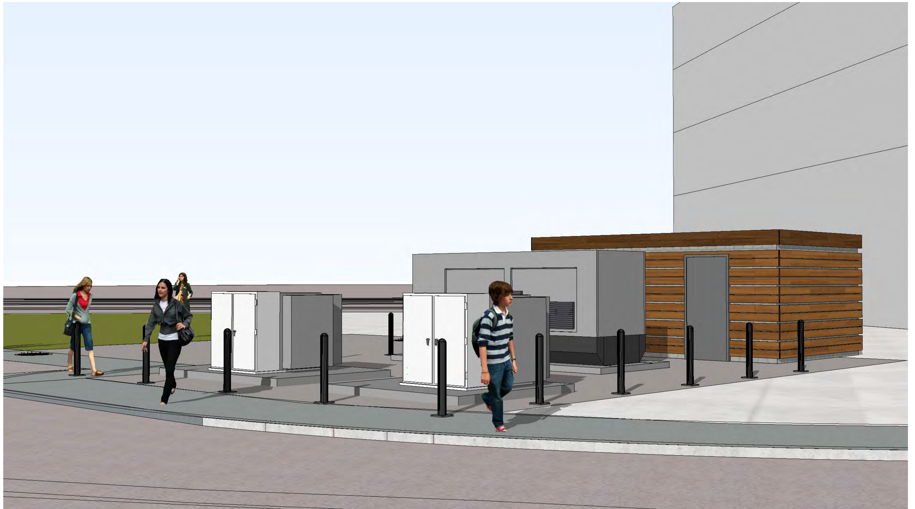
Wood clad pump station building with no fence & trellis
