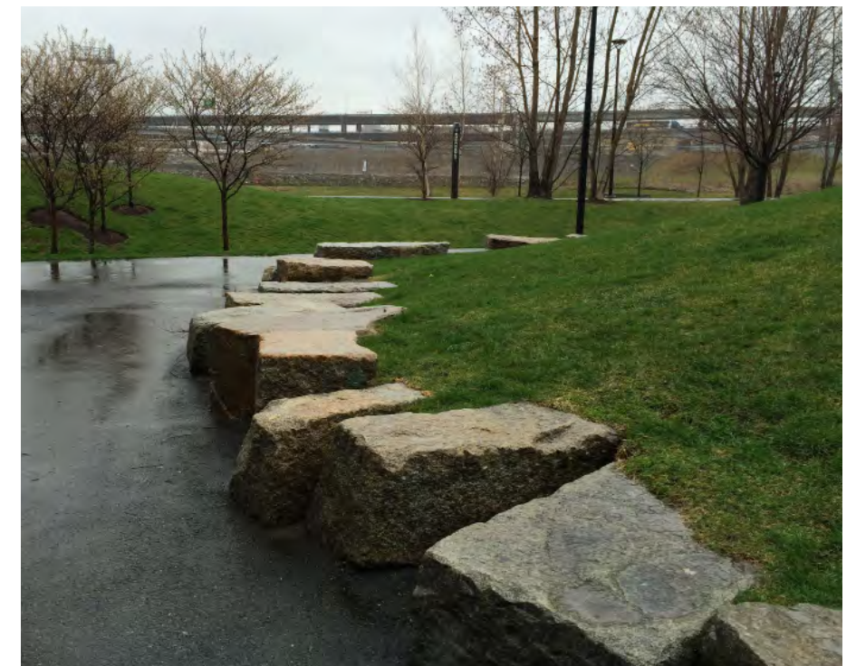
Reclaimed Granite Block Seatwalls
