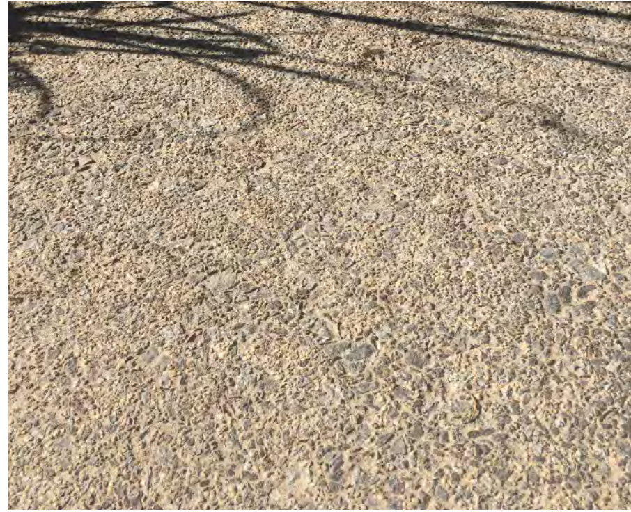
Exposed Aggregate Concrete Pavement
