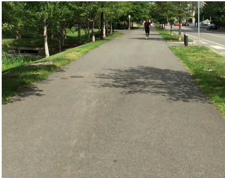
Bituminous Concrete Pavement
