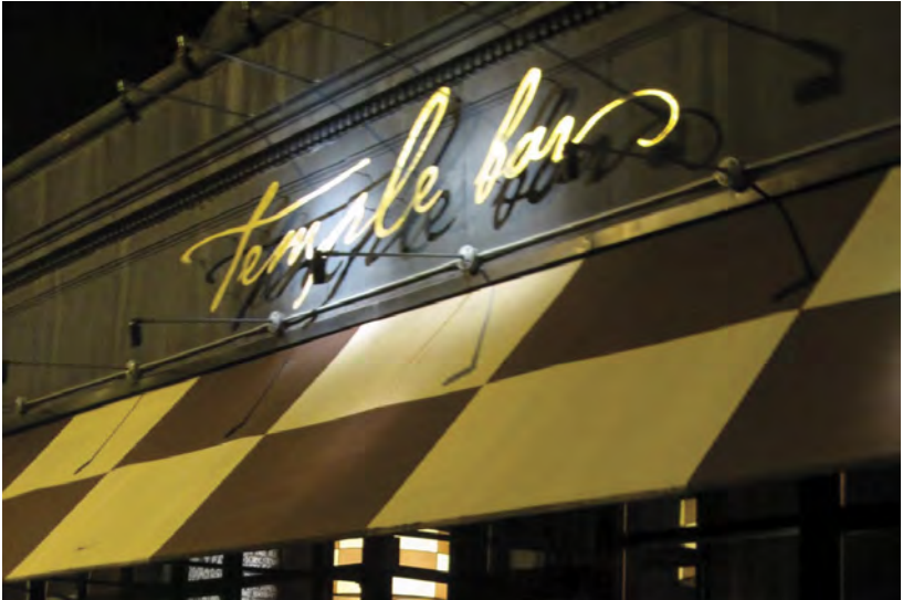
Preferred: Exterior gooseneck-type lighting of individual lettering. Continuous strip lighting is not allowed.
