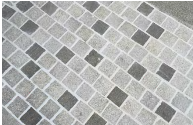
Stone Setts Pavement
