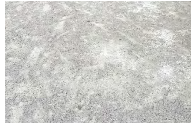
Decomposed Granite Pavement
