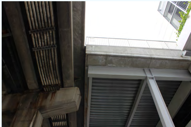
Gilmore Bridge, Existing Condition
