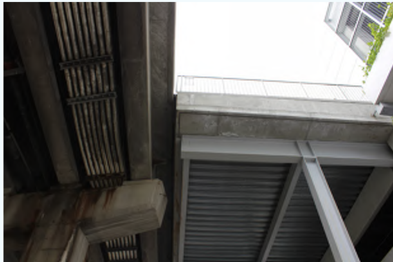
Gilmore Bridge, Existing Condition
