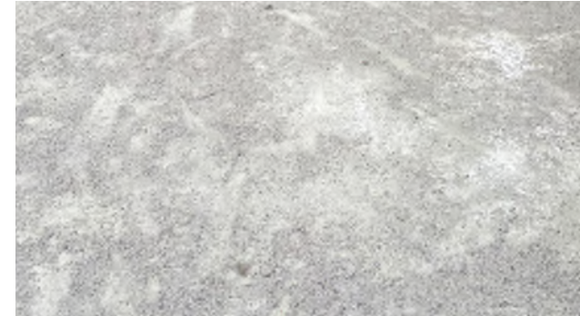
Decomposed Granite Pavement
