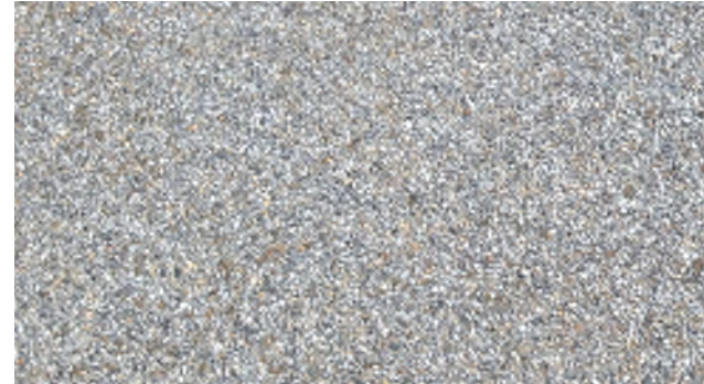
Exposed Aggregate Concrete Pavement
