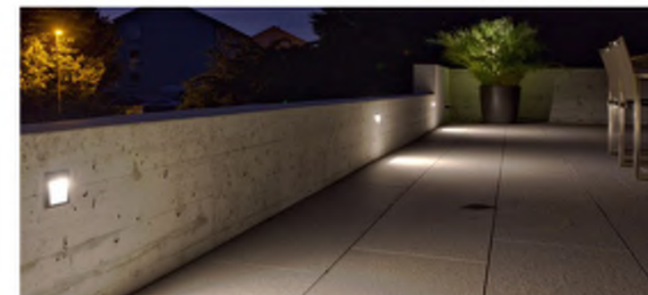
5 Step Lighting in Curb
