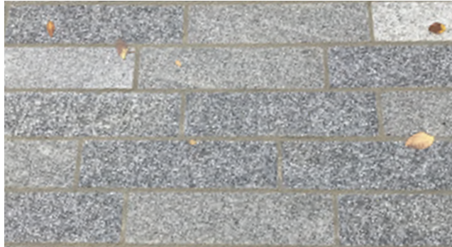
Stone Setts Pavement
